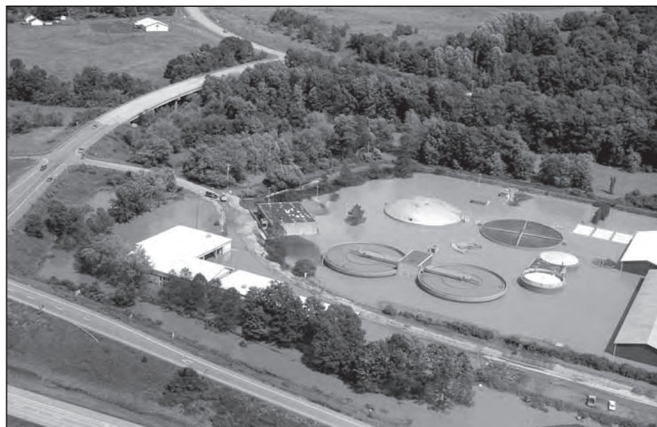
The Oneonta WWTP inundated by the June floodwaters
