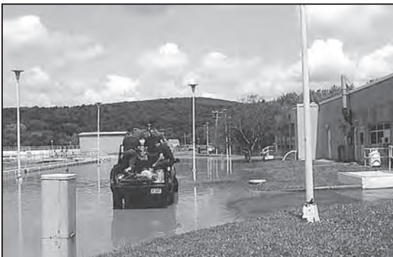
Plant personnel evacuated after safeguarding equipment and turning the power off.
