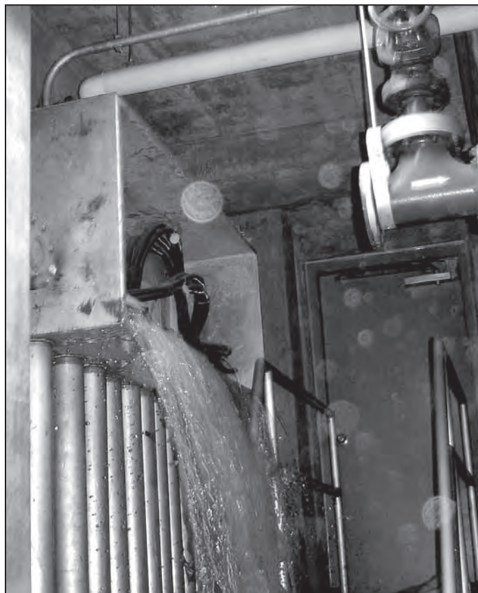
Water pours into a basement area via existing electrical conduits and junction box.
