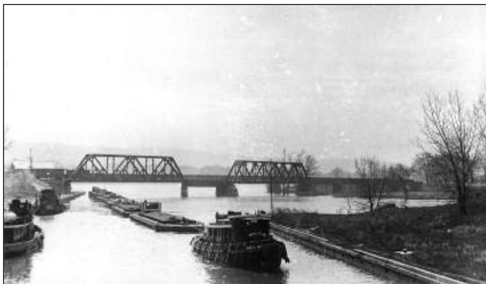
Tug tows a fleet of barges toward Lock E-2 on the new Barge Canal
