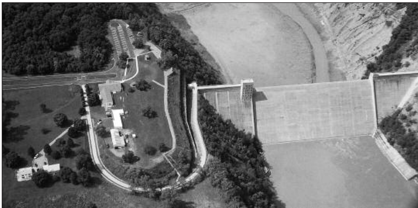
Mt. Morris Dam, the largest concrete dam east of the Mississippi, as seen by air
