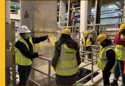
2022's InFLOW participants tour NYC's Newtown Creek Water Resource Recovery Facility (WRRF) with Pam Elardo, Deputy Commissioner, Bureau of Wastewater Treatment New York City Department of Environmental Protection.
