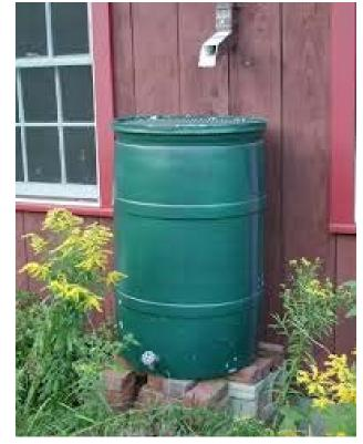
Rain barrels capture rain runoff from a building's roof using the gutter and downspout system. Rain barrels help reduce pollutants and the velocity of water entering local rivers and streams.
