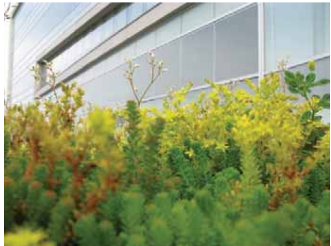
This green roof on the Syracuse Center of Excellence retains stormwater, effectively increasing system capacity.
