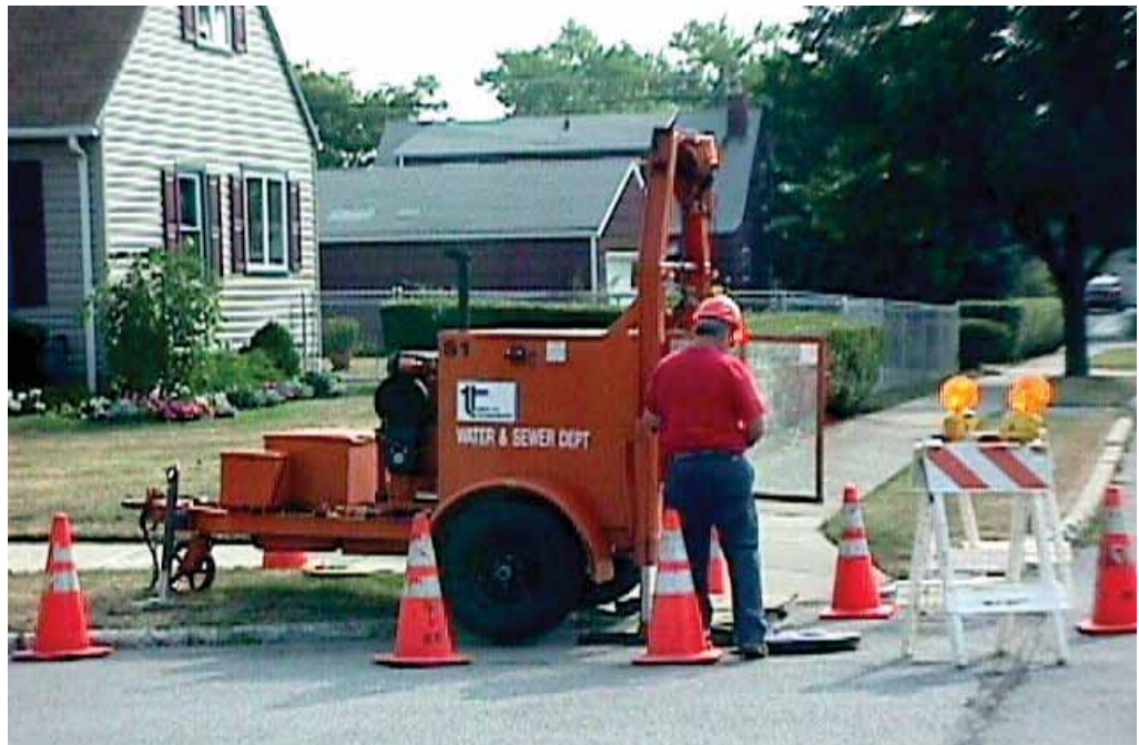
Proper maintenance of the collection system is critical for optimum system performance. (Town of Tonawanda).
