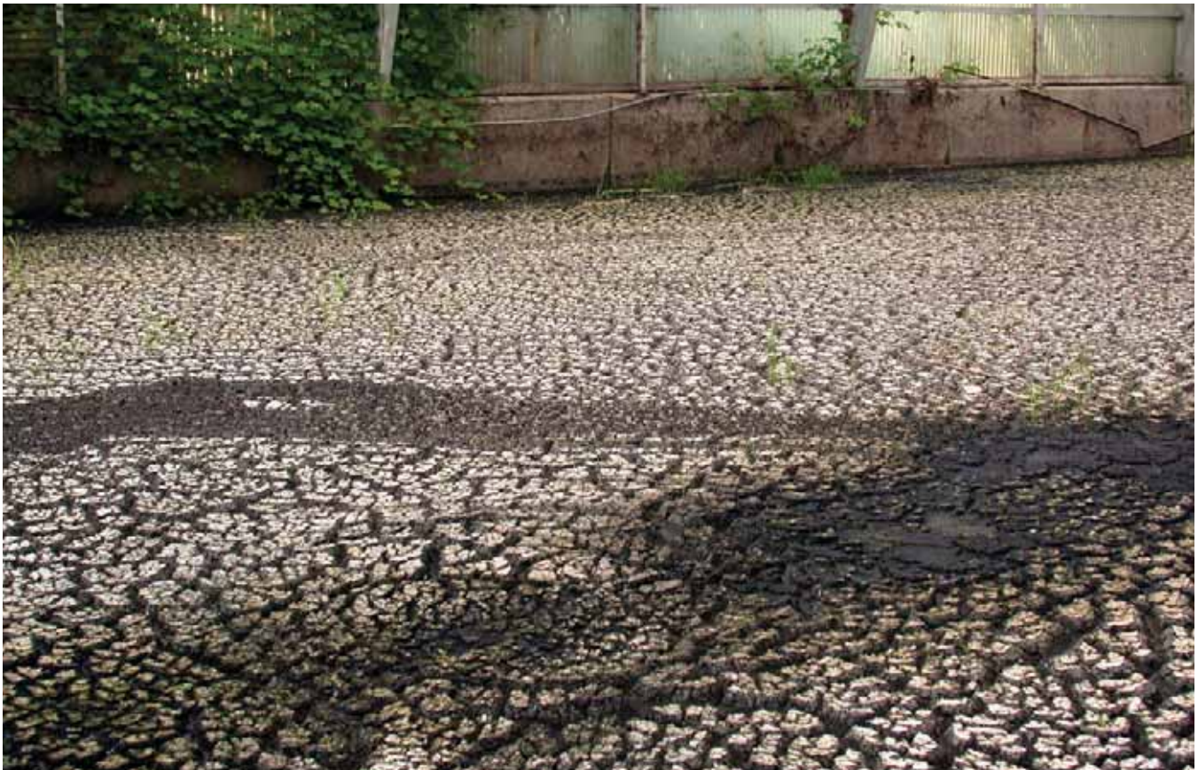
Sand drying beds can be problematic, particularly with rainy conditions.
