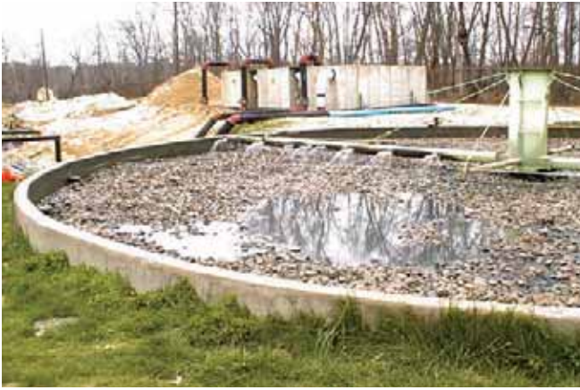
Fixed film and old trickling filter stone, left, are sometimes replaced with more efficient plastic media, right.
