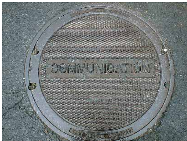
As stamped on the manhole cover above, communication is at the heart of good management.
