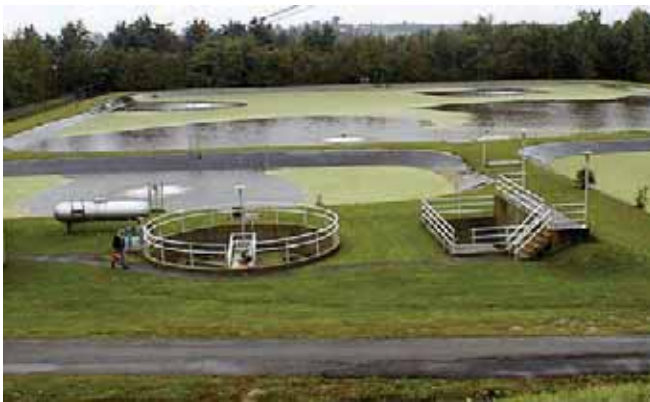
Aerated lagoons are secondary treatment processes.
