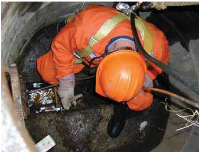
Confined space training is necessary for linear asset maintenance.
