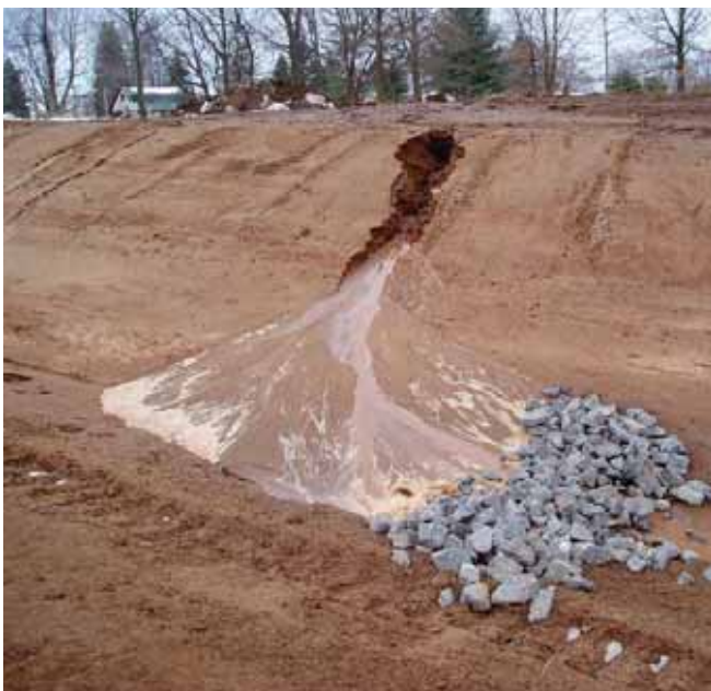
A minimum number of controls is necessary during construction.
