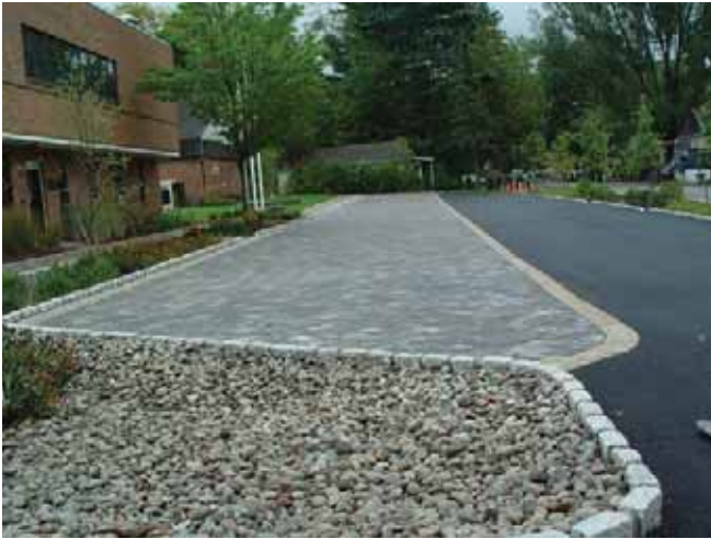
Porous pavers, and bioswales adjacent to the municipal building in the Village of Greenwood Lake provide a visible demonstration project. Project funded by the Green Innovation Grant Program. Photo credits: NYS EFC.
