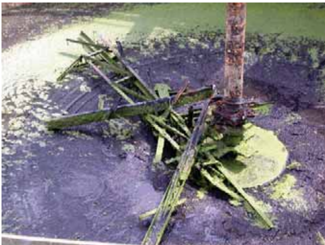
Sometimes repair is not possible and equipment must be replaced. Good maintenance strategies can prevent catastrophic failure.
