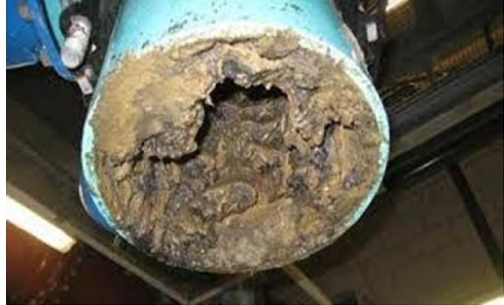
**Fats, Oils, and Greases** should not go down drains. Over time it will get hard and clog pipes. If wastewater can't move through the pipes it can cause flooding, sewage to backup in your home, and issues at wastewater treatment facilities. To dispose of this material wait until it cools down and throw it away in a nonrecyclable container.
