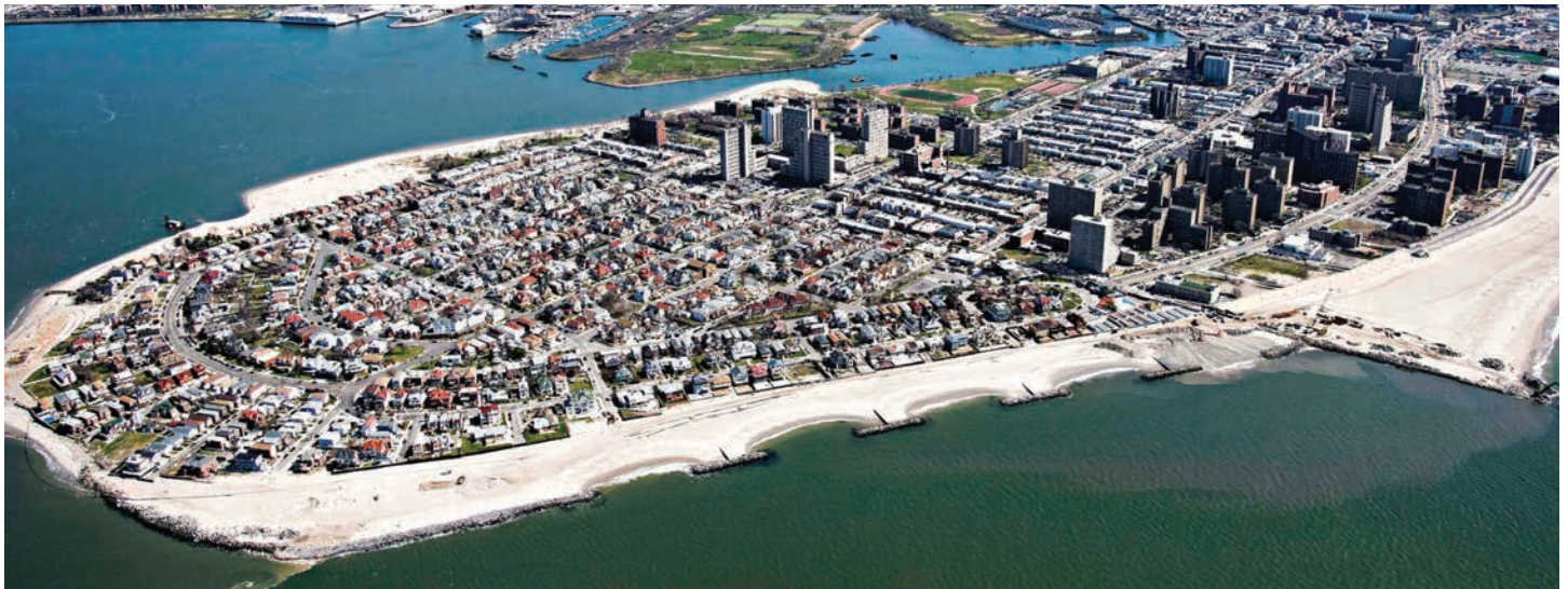
Aerial image of the Sea Gate portion of the Coney Island peninsula showing the completed T-groins in 2016.
