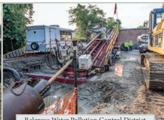
Belgrave Water Pollution Control District
