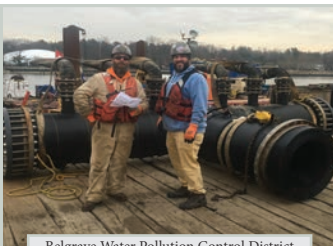
Belgrave Water Pollution Control District
