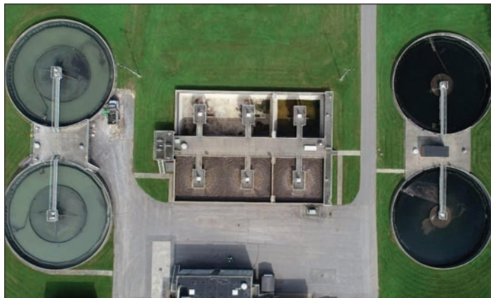
Overhead view of the Herkimer County Sewer District WWTP with primary settling tanks (left), aeration tanks (center) and final settling tanks (right).
