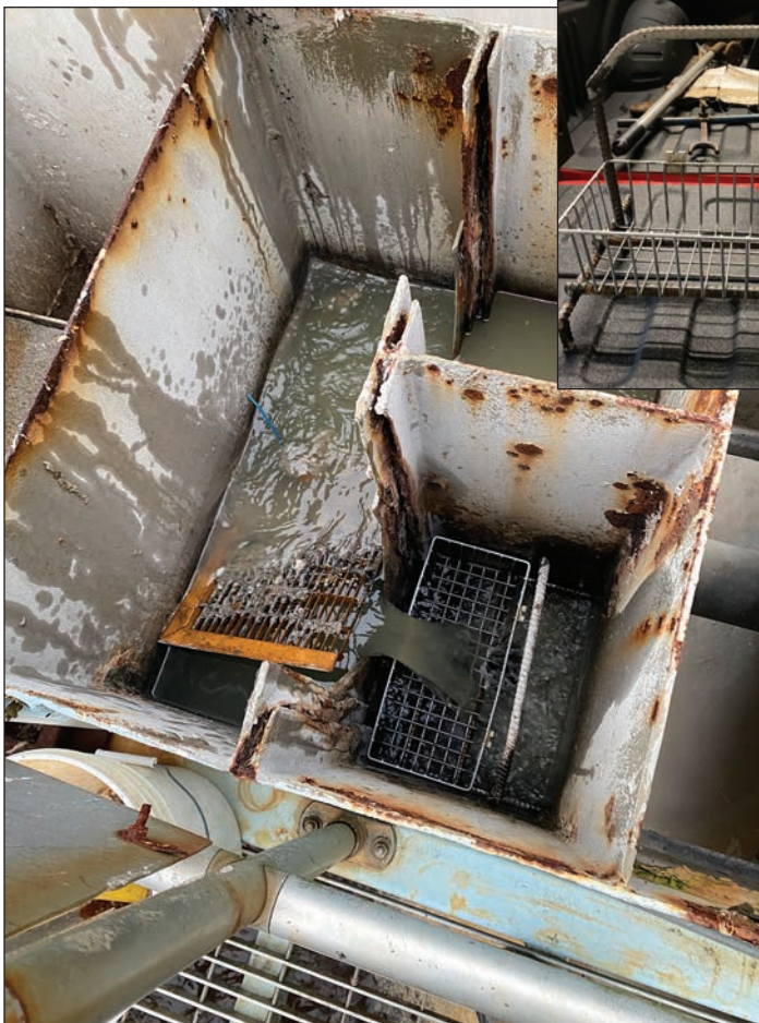
DIY rag collection project (inset) in the headworks. David Hinds
