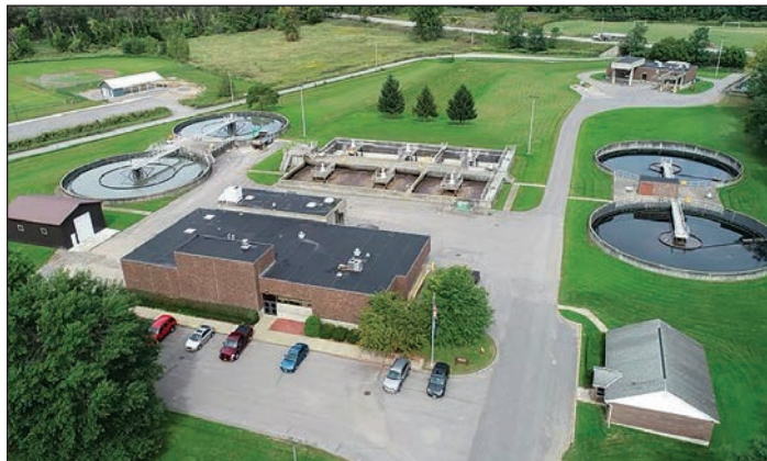
Birdseye view of the Herkimer County Sewer District WWTP showing the pump station (upper right), the District Office (lower right) and a storage barn (center left). Chlorine contact tanks are barely visible in the upper right corner adjacent to the pump station.
