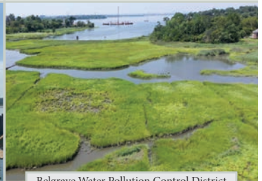
Belgrave Water Pollution Control District
