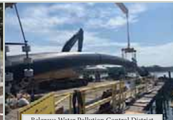
Belgrave Water Pollution Control District
