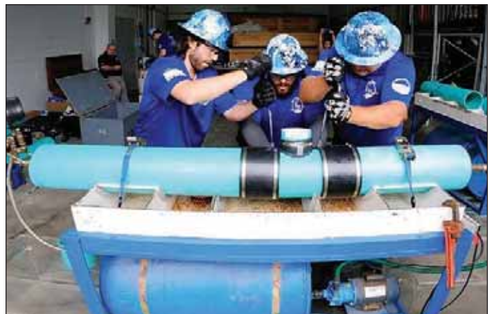
Team members fastening tension bands on Fernco to ensure a seal.
