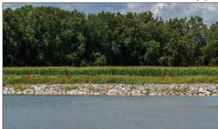
Before (left) and after (right): Edelweiss Property streambank restoration project using rock riprap. This project stabilized 1,980 linear feet of un-buffered agricultural field along the west bank of the Genesee River in the Town of Hume, New York. It reduced sediment and phosphorus loads to the river by adding a new riparian zone while emphasizing the use of bioengineering techniques and habitat enhancement. Stabilization of the riverbank and the establishment of a vegetated buffer on the reduced bank slope has significantly reduced the rate of erosion and the subsequent loss of agricultural land. (Source: Genesee RiverWatch).
