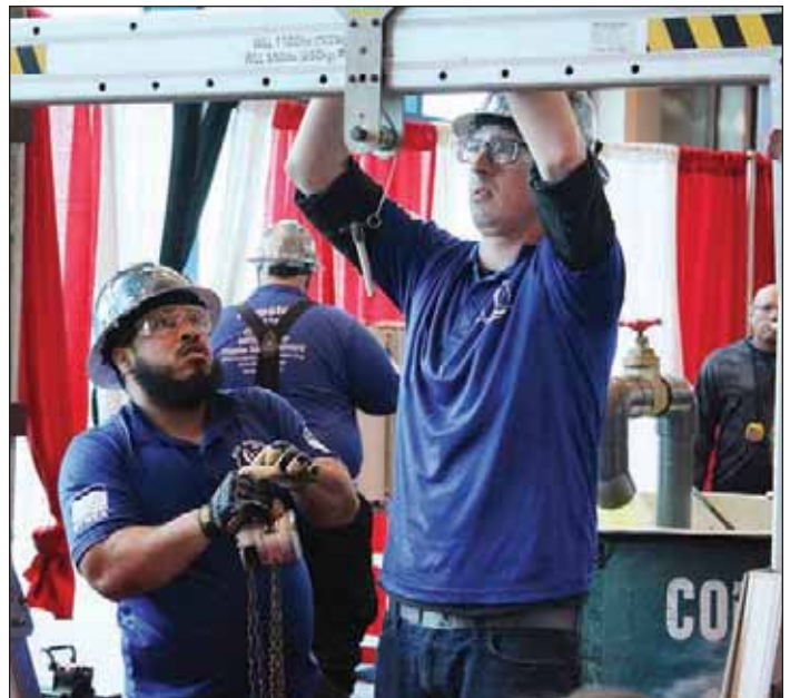
Team members prepare the gantry unit for pump removal.
