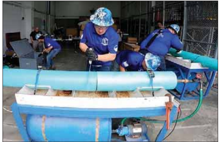
Team members cutting PVC pipe during collections event.
