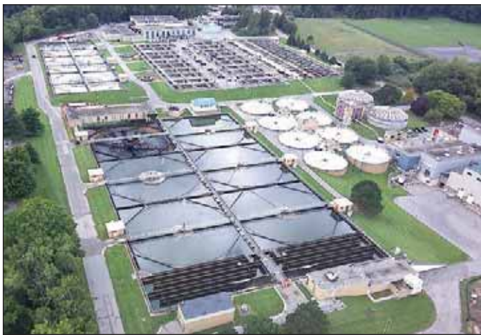
Aerial image of the Van Lare WRRF, September 2022.
