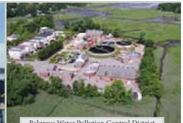
Belgrave Water Pollution Control District
