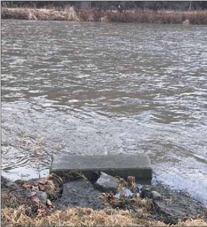
The Village of Bath WWTP outfall discharges to the Cohocton River.
