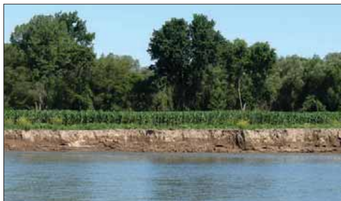
Before (left) and after (right): Edelweiss Property streambank restoration project using rock riprap. This project stabilized 1,980 linear feet of un-buffered agricultural field along the west bank of the Genesee River in the Town of Hume, New York. It reduced sediment and phosphorus loads to the river by adding a new riparian zone while emphasizing the use of bioengineering techniques and habitat enhancement. Stabilization of the riverbank and the establishment of a vegetated buffer on the reduced bank slope has significantly reduced the rate of erosion and the subsequent loss of agricultural land. (Source: Genesee RiverWatch).
