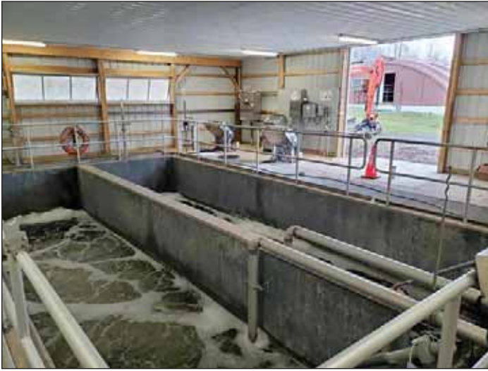
WCWSA UV Disinfection Project at Eastern Regional WWTP. WCWSA
