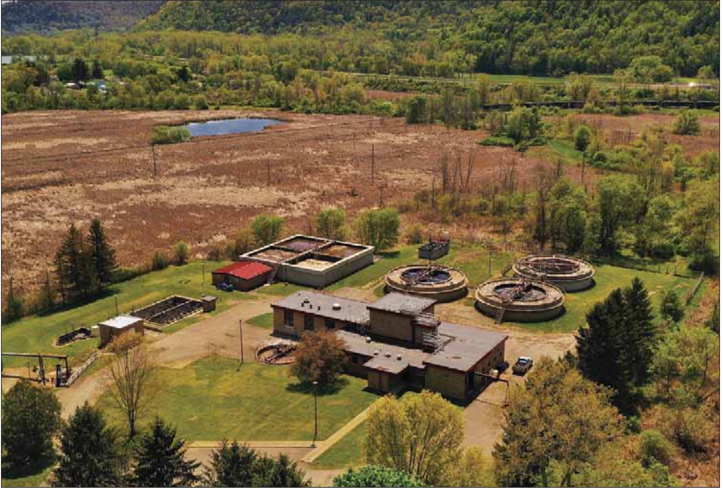
Aerial view of the Village of Bath WWTP.
