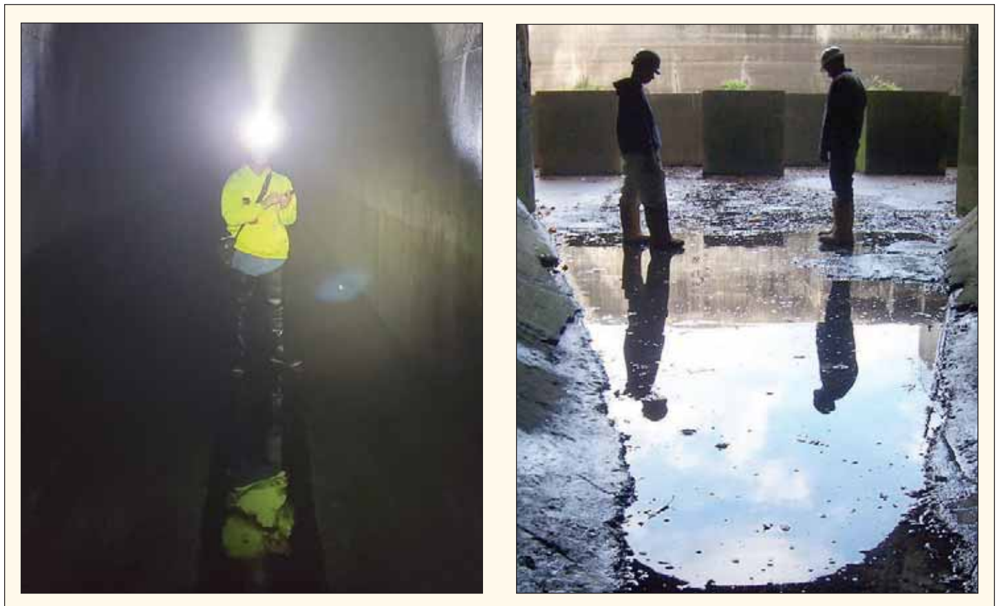
Inspecting the CSOAP Tunnels.
