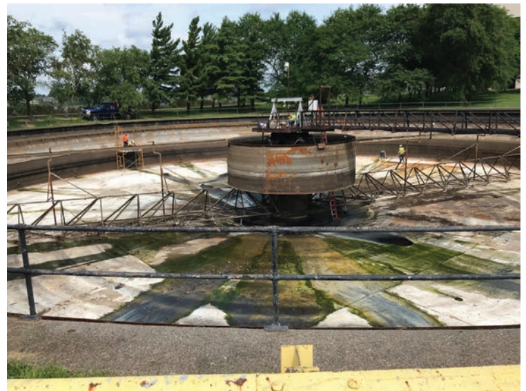
Figure 13. Primary tank inspection.
