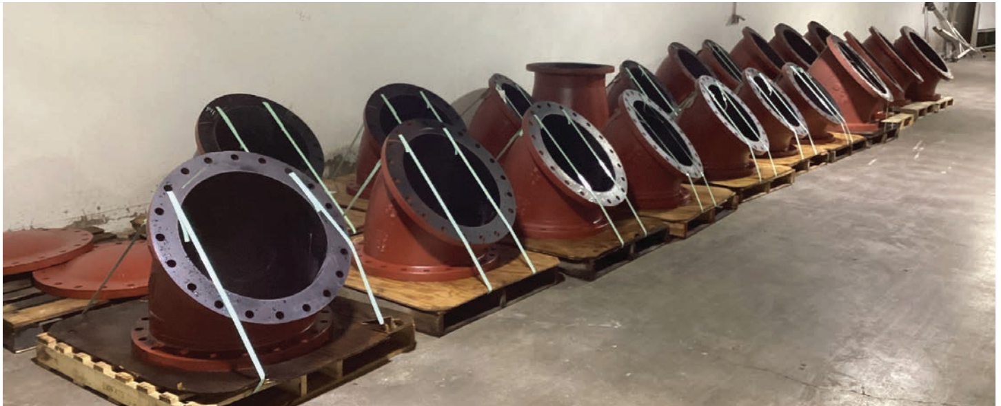
Figure 11. Bird Island WWTF large diameter ductile iron pipe fittings staged for installation. AECOM
