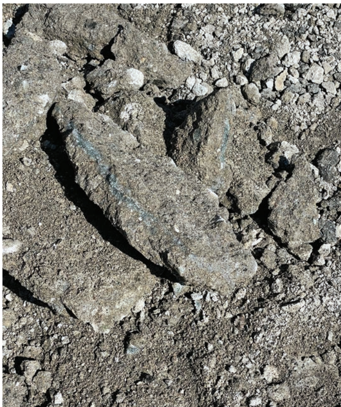
Teal and bright green lines found in what was thought to be a concrete road base that turned out to be slag TENORM. Casterland Fanfan
