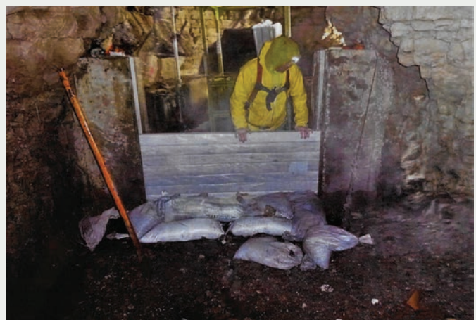
Inspecting a new tunnel regulator diversion dam.
