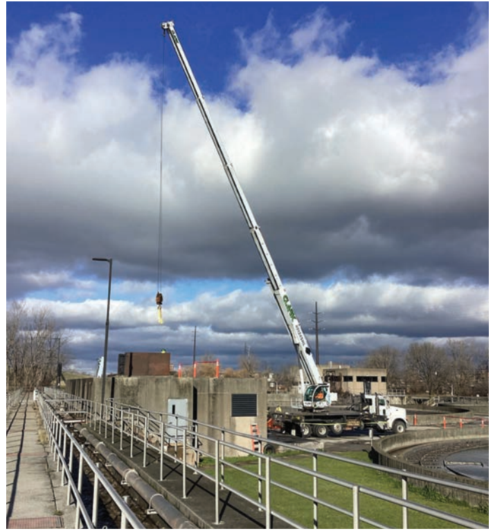
Figure 10. Bird Island WWTF large diameter ductile iron pipe delivery. AECOM
