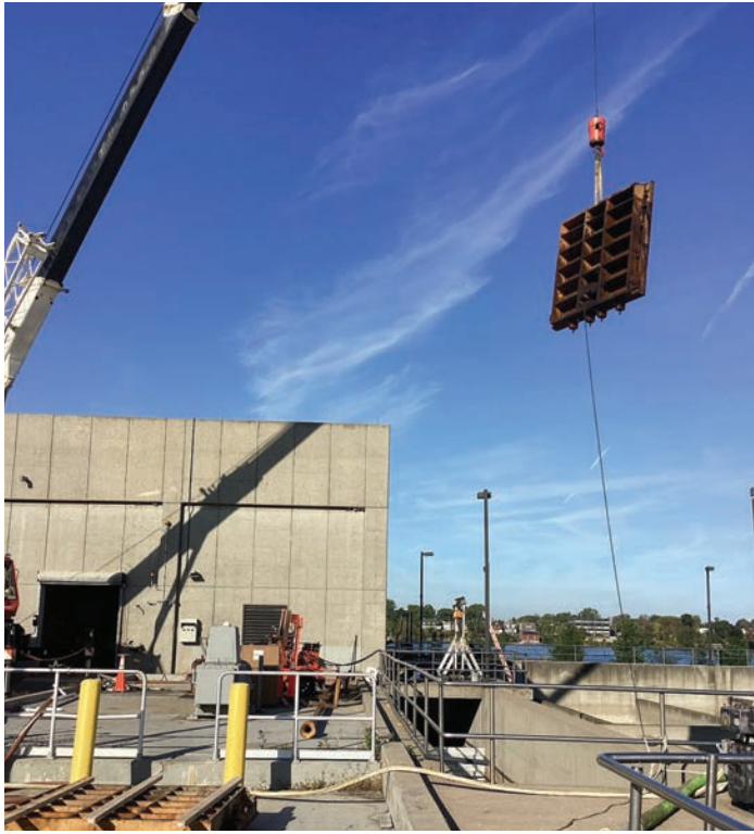
Figure 9. Bird Island WWTF chlorine contact tank sluice gates during removal. AECOM
