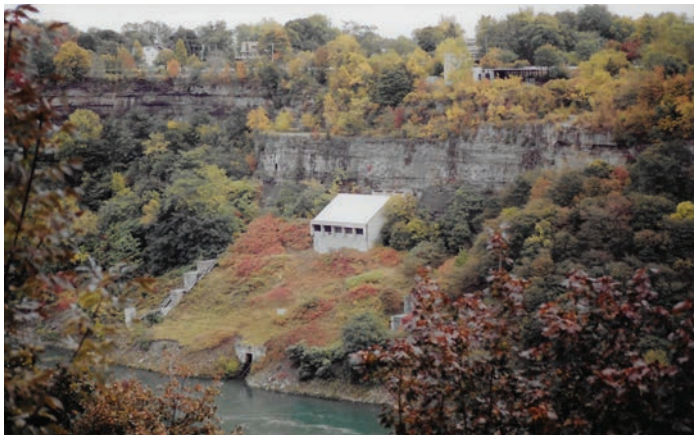
Figure 3. Gorge Pumping Station can be seen from Ontario, Canada, looking northeast across the Niagara River. Rick Roll
