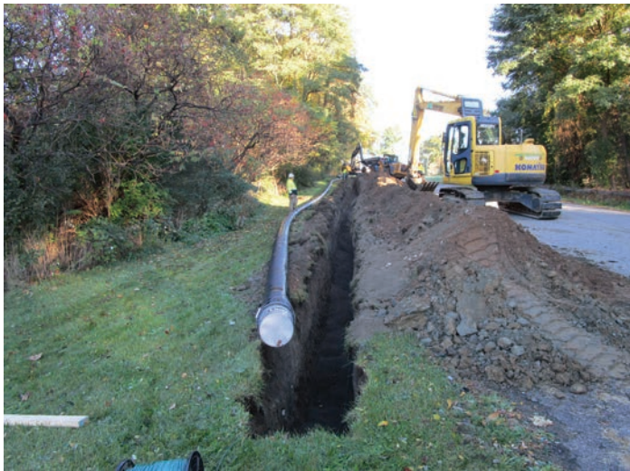
Main line sewer installation.
