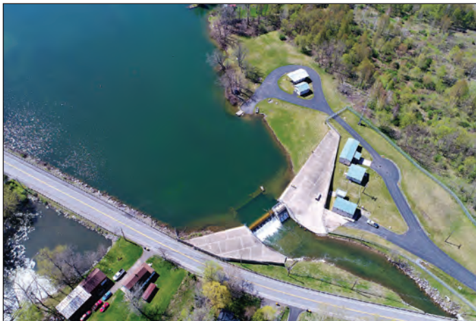
Aerial view of the Otisco Lake Dam in 2017, after completion of the rehabilitation project OCWA
