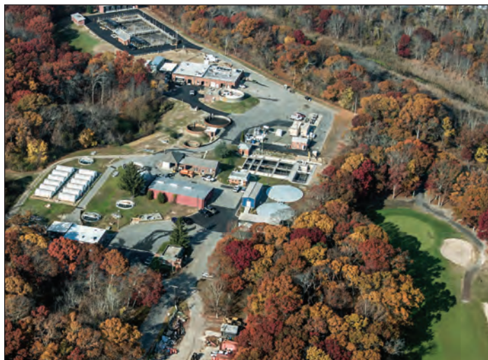
Post-construction aerial view of the Riverhead Water Resource Recovery Facility and Indian Island Golf Course. H2M architects + engineers
