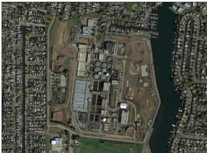
Figure 2. Bay Park Sewage Treatment Plant. Nassau County
