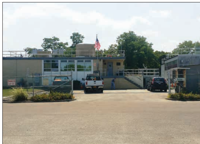
The Village of Northport made significant upgrades to its water resource recovery facility. Tony Lopez Photo
