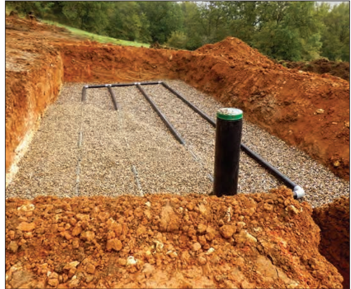
Septic sand and gravel drainage system. Septic systems are common in the northern portion of Nassau County. istockphoto.com
