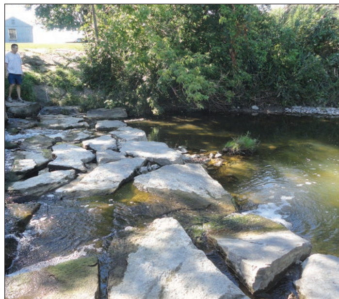
Photograph 1. Pre-construction view of the Tarbell Road habitat restoration site on the South Branch of Ley Creek. Les Monostory
