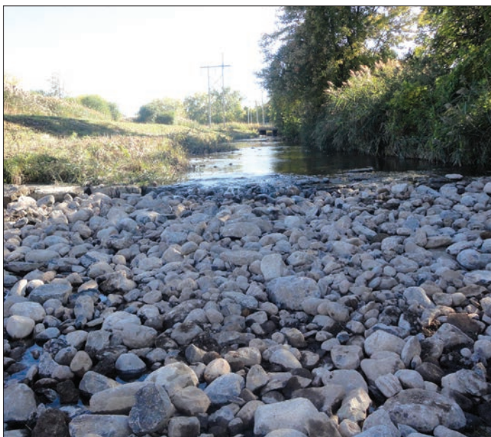
Photograph 3. The stone fill is placed in the streambed at the site of the stone dam structure and downstream. The creek's water is flowing through the voids under the stone fill.
