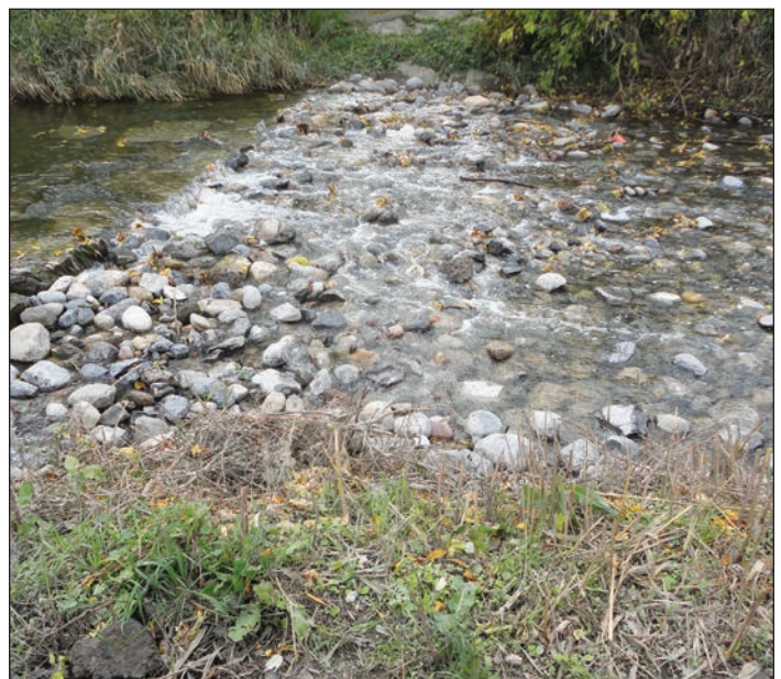
Photograph 4. One week post-construction, heavy rainfall raised the water level of the South Branch of Ley Creek, allowing for the deposition of silt and mud in the gaps between the stones so the stream flowed across the top of the fill.
