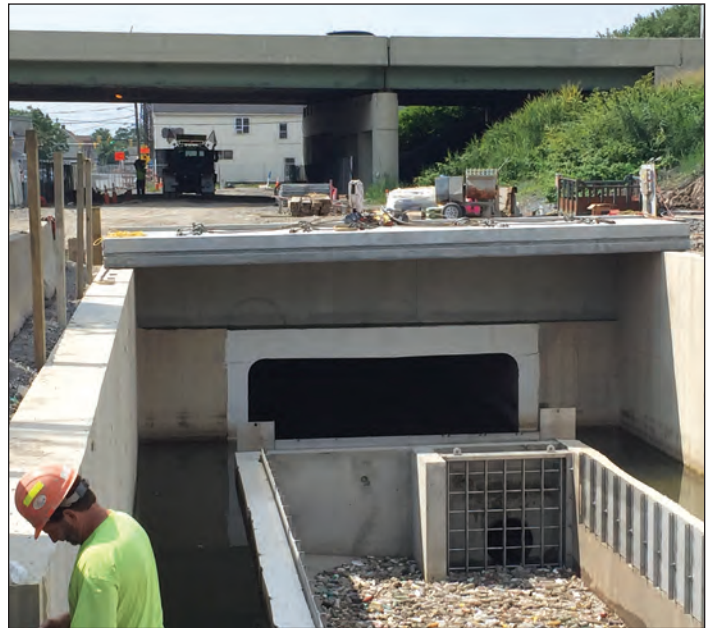
Figure 10. Smith Street RTC under construction. GHD and J.M. Davidson
