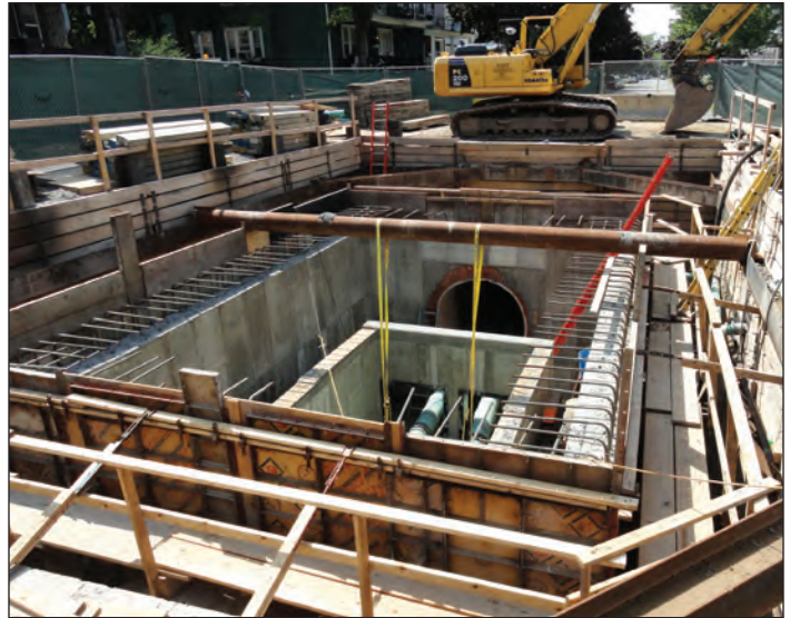
Figure 4. Construction of the Bird Avenue RTC underway. GHD
