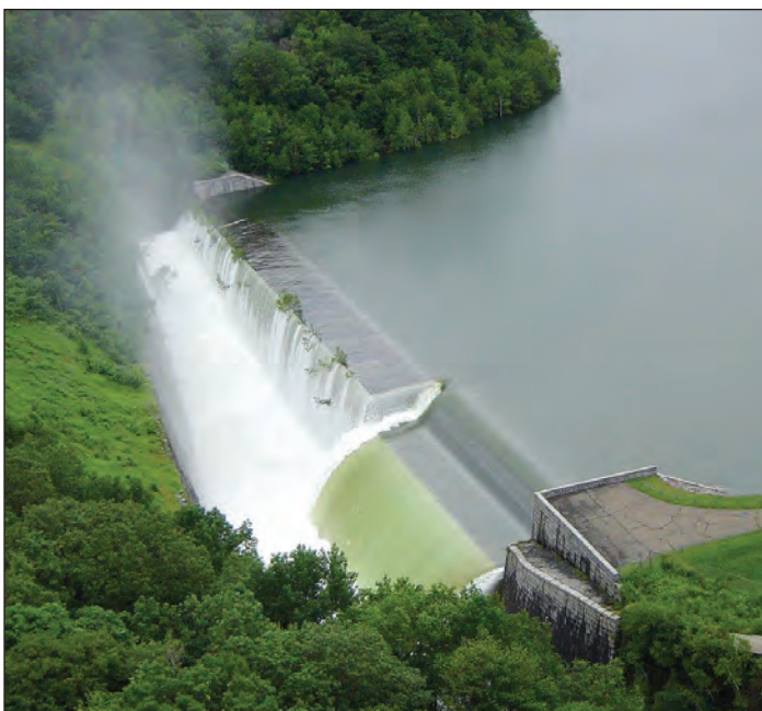
Cannonsville Spillway. NYCDEP
