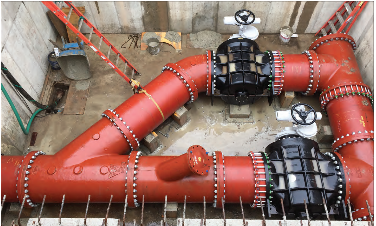
Figure 11: Smith Street RTC large valve pit under construction.
