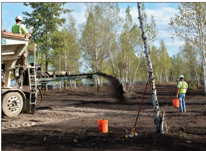
OCRRRA compost was applied at a rate of 300 cubic yards per acre.
