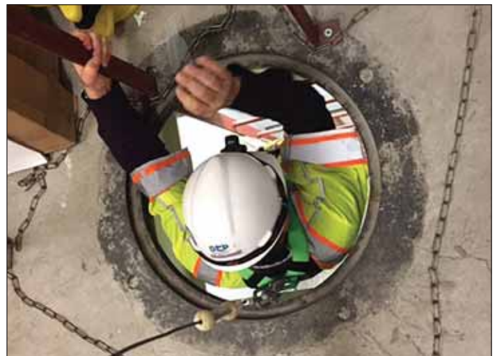
An Apprentice Construction Laborer learns how to safely enter a confined space.
