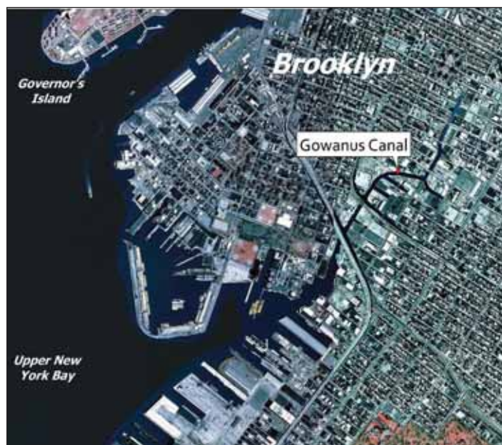
Figure 1. Orthoimage of the Gowanus Canal and surrounding terrain in the borough of Brooklyn, New York.
