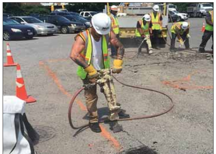
Safe operation techniques for using a jackhammer are practiced by an Apprentice Construction Laborer.
