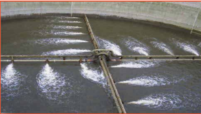
JET MIXING IN EQUALIZATION TANKS
