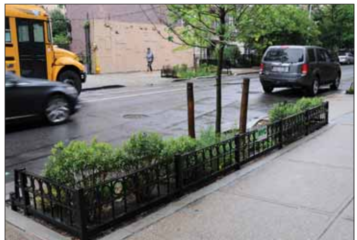
Bioswales are one of the green infrastructure assets that have been implemented throughout the city for control of stormwater runoff.
