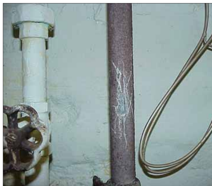
A simple scratch test can tell you if your line is lead. Madison Water Utility
