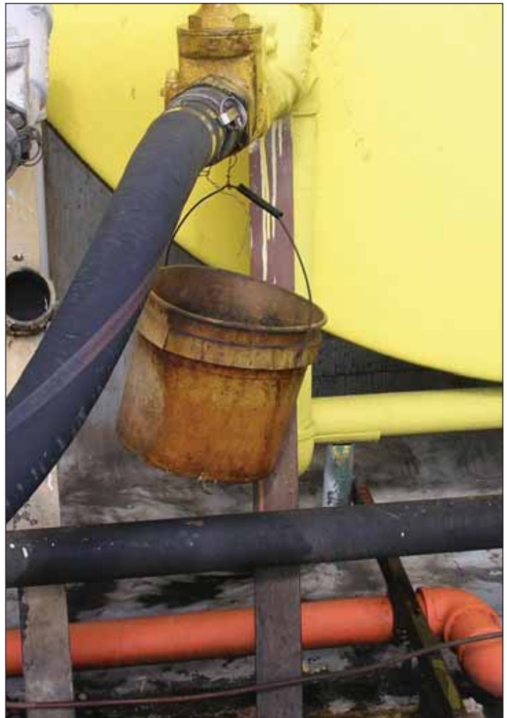
This "solution" may be an indication of generally weak maintenance practices and the potential for releases to the environment.
