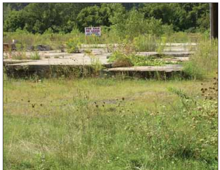
Validate indications of former structures against maps of known site structures and their past uses. OBG
