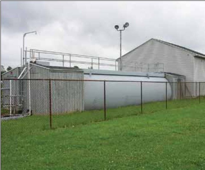
Where there is no daylight between bulk storage units (of any kind) and the ground, tank condition cannot be visually assessed.
