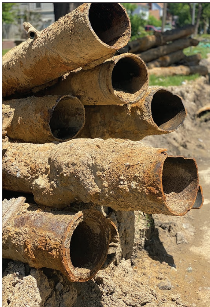
Lead pipe removal in Flint, MI.
