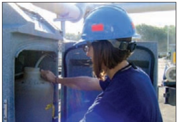
Alison Perez, a Pump and Process Operator trainee, checks an automatic sampler at the VanLare WWTP in Rochester, NY.
