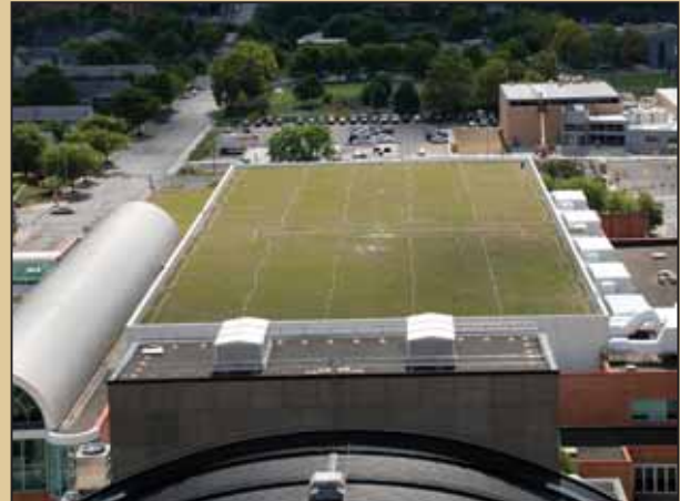
Green roof at Oncenter's Nicholas J. Pirro Convention Center
