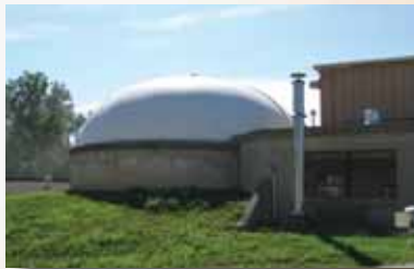
Digester Gas Holding Cover
