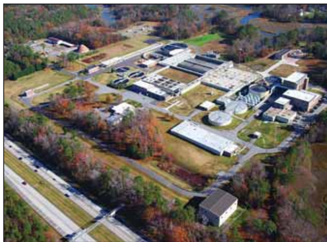
Figure 1: Nansemond Treatment Plant in Suffolk, VA.
