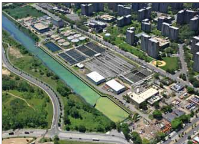
An aerial view of the 26th Ward WWTP located in Brooklyn, with Jamaica Bay in the background. The newly built and first-in-the-nation separate centrate treatment (SCT) wastewater facility that operates a glycerol storage-and-feed system is reducing effluent nitrogen by 67 percent.
