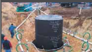
Courthouse Commons Pump Station
