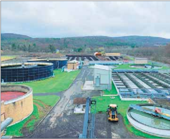
Village of Endicott WWTP showing gravity thickener, anaerobic digester, primary clarifiers, biotowers, secondary clarifiers and windrow compost. Philip Grayson
