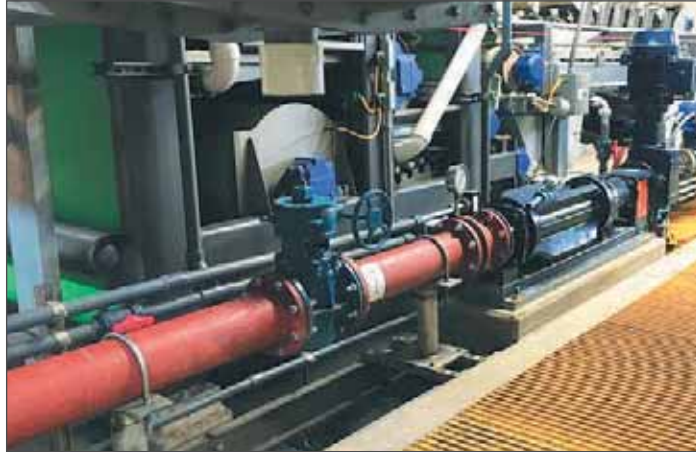
The Rome WRRF recuperative thickening return pump. George Bevington, B&L
