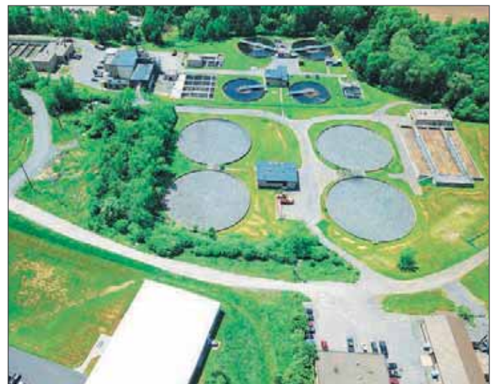
City of Auburn Water Pollution Control Plant. The decommissioned trickling filters and recirculation building in the center of the image will be the location of the digesters, dryer building and product storage barn.
