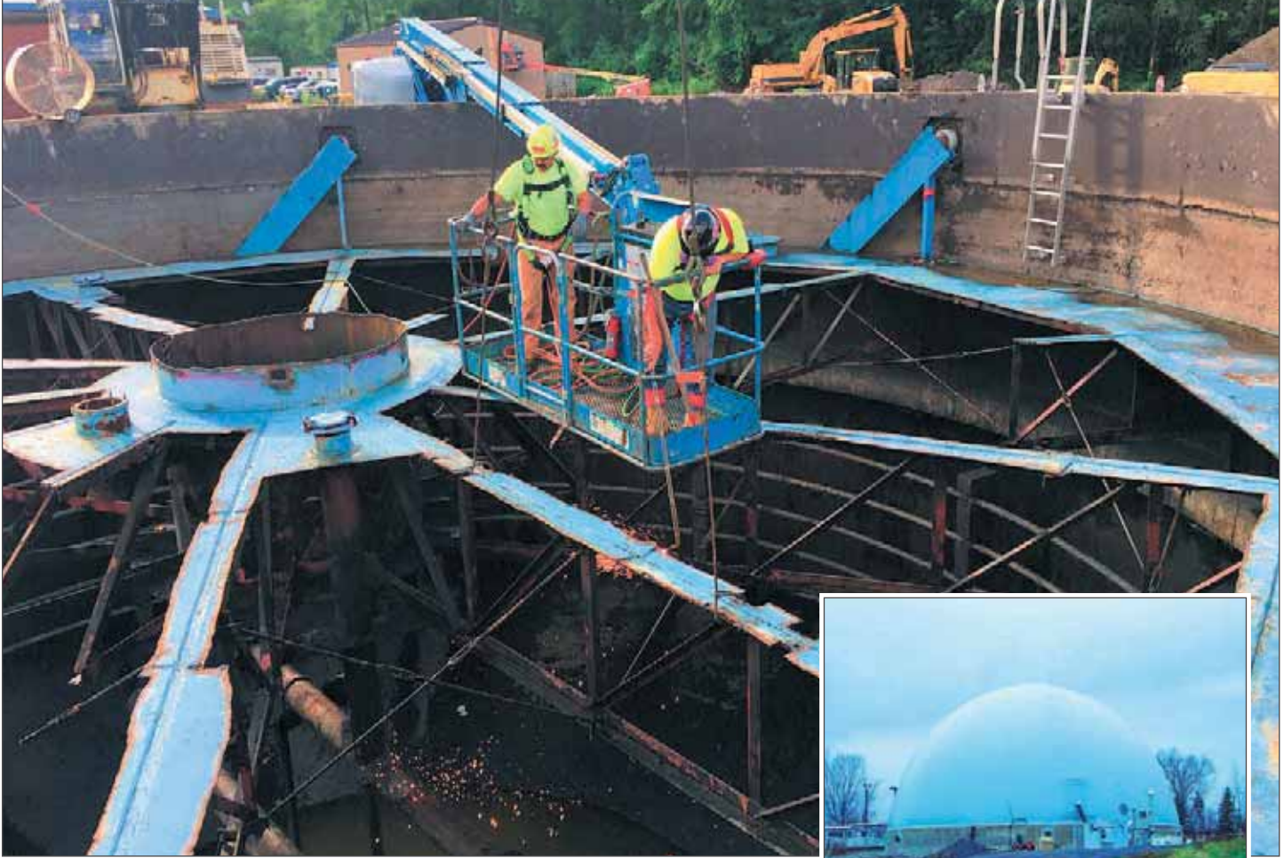
Demolition of Digester 2 Cover. George Bevington/B&L
