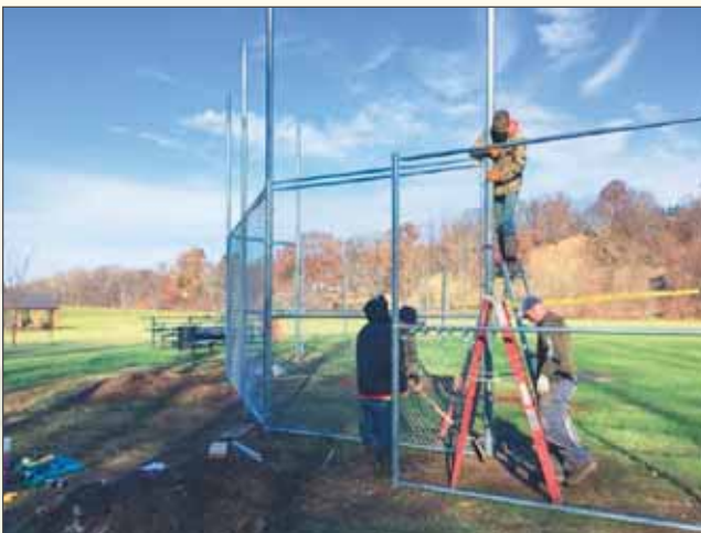
Baseball field construction.
