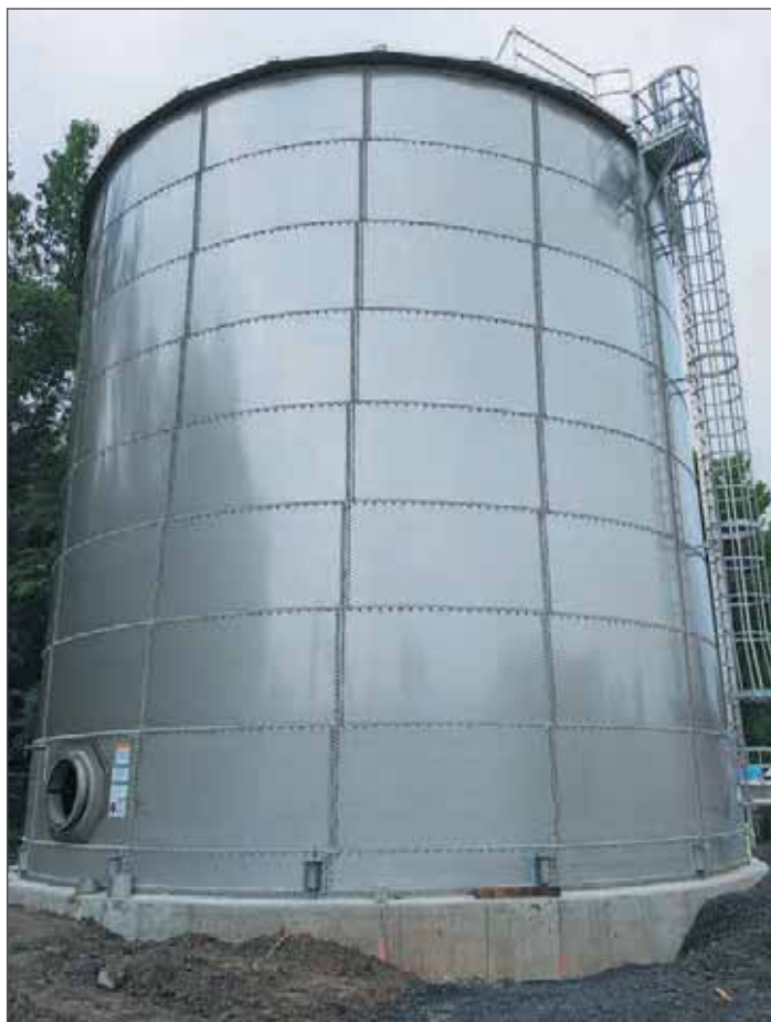
HSOW stainless steel equalization tank.
