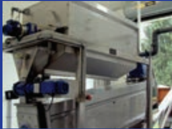
Groton NY WWTP Model 3012 DSP Screw Press
