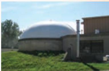
Digester Gas Holding Cover
