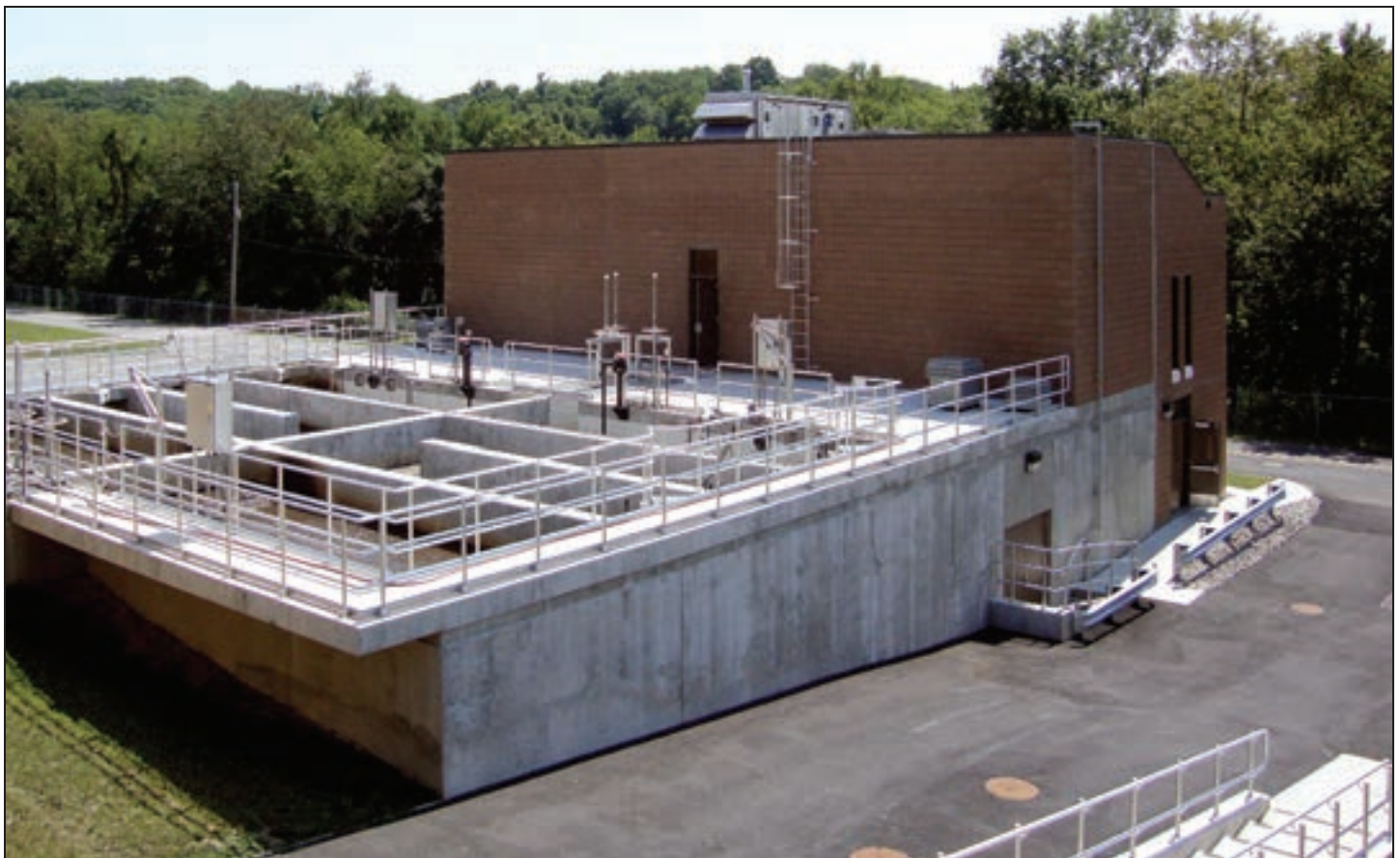
Figure 4. This shows a plant designed for biological nutrient removal limits and cold weather operation (influent temperature is 8 degrees Celsius). Its hydraulic capacity is 265,000 GPD and the effluent from the plant is recycled. This design has process tanks outside and equipment inside with a footprint of 59-by-54 feet for the process tanks.
