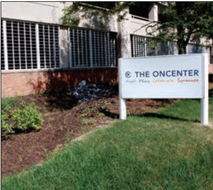
Rain gardens at Oncenter Municipal Parking Garage
