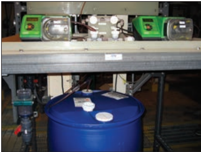
The catalase enzyme is fed to the system through this tank at a rate of less than 0.02 gallons per hour.
