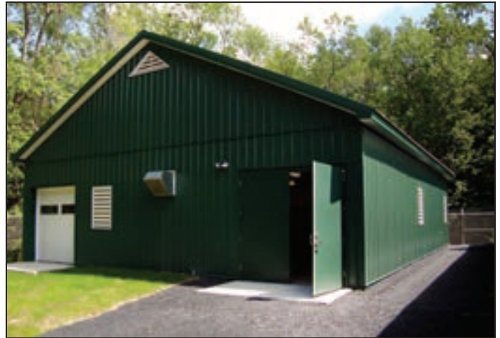
Figure 3. This 90,000 GPD MBR plant fits into a 48-by-36-foot building. This building includes the fine screens, process tanks, control room generator set and all equipment, enclosing the entire plant.
