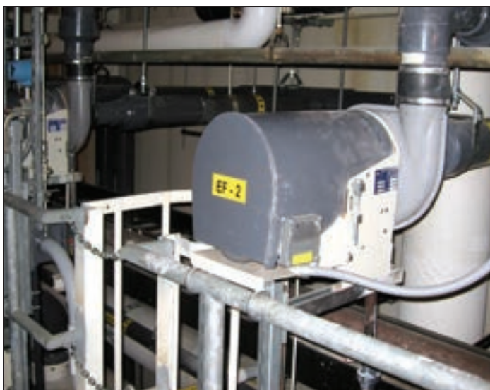
Two new fans carry oxygen away from the reaction tanks to avoid accumulation of oxygen within the treatment system.
