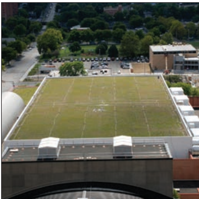
Green roof at Oncenter's Nicholas J. Pirro Convention Center
