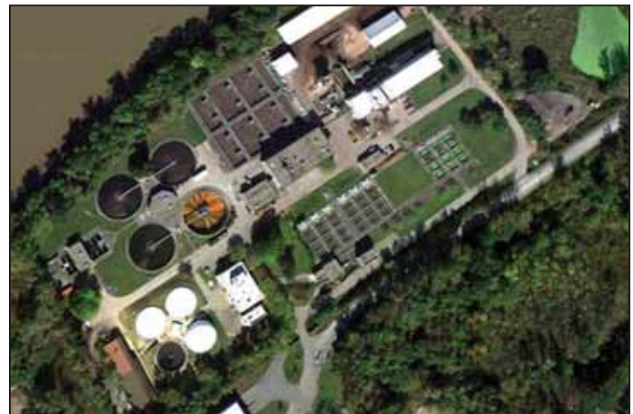
Figure 2. Aerial view of Schenectady's Water Pollution Control Plant
