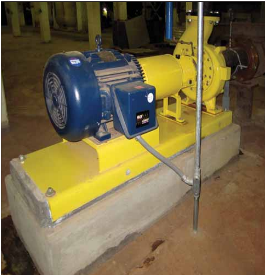
Pumps typically consume large quantities of energy. Consider installing premium efficiency motors and variable frequency drives (VFDs), or re-sizing the pumping system.
