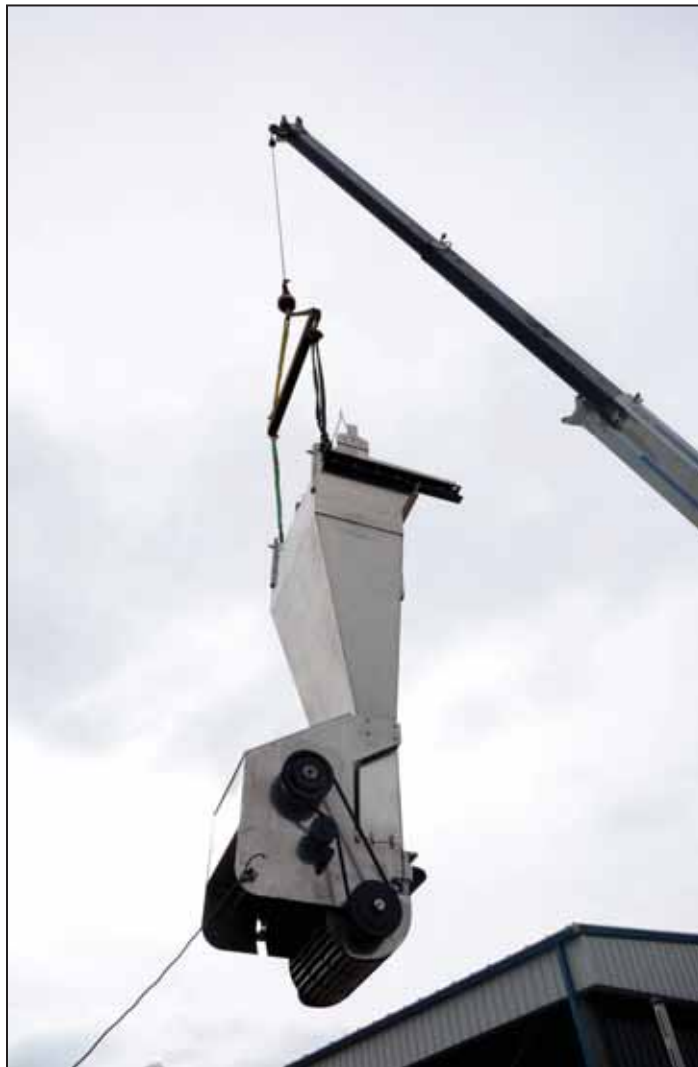
Figure 4. The cross-flow turbine engine being lifted into place
