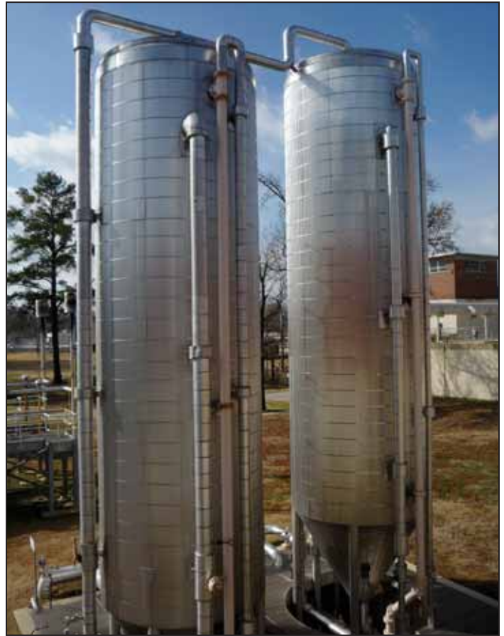
New anaerobic digester process – Columbus (GA) biosolids flow through thermophilic treatment Anaerobic Digestion (Biodegradation Pathway).
