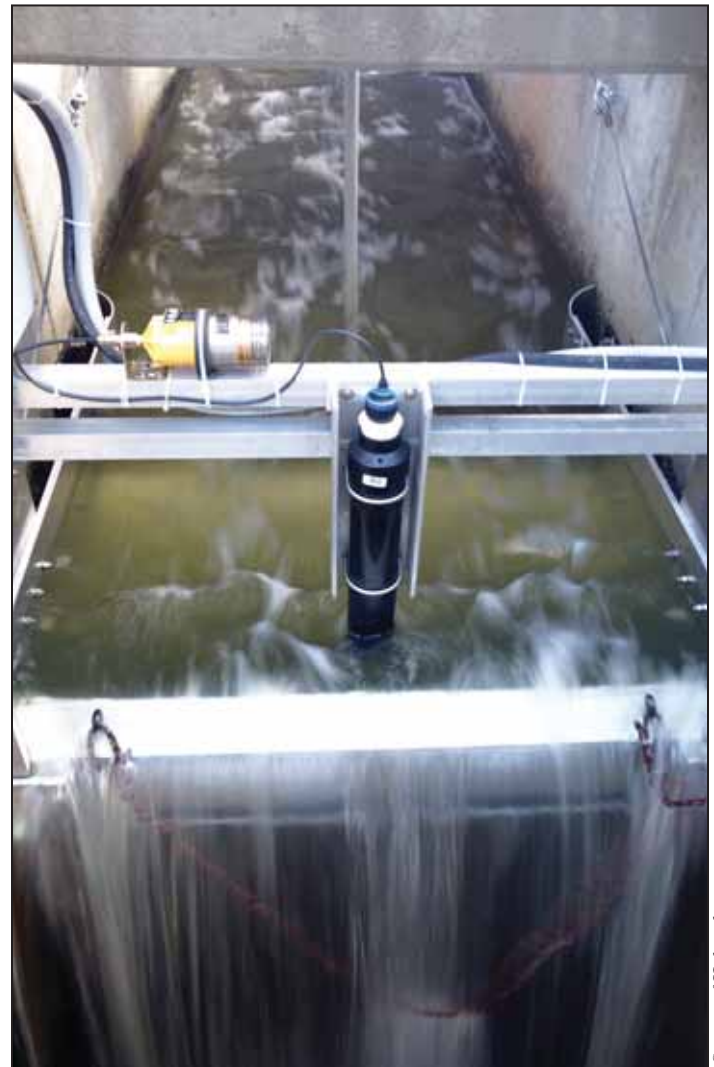
Figure 5. Shown in operation, the turbine generates electricity through the outflow.
