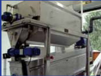
Groton NY WWTP Model 3012 DSP Screw Press
