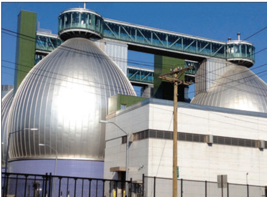
The NYC Department of Environmental Protection spent $5 billion to upgrade its largest wastewater treatment plant, Newtown Creek, which has 310 mgd treatment capacity (this shows a section of the plant's iconic egg-shaped digesters). Long-term bond issuances were acquired by NYCDEP's financing arm, the NYC Water Finance Authority, to finance this, among other major projects.
