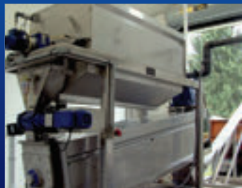
Groton NY WWTP Model 3012 DSP Screw Press
