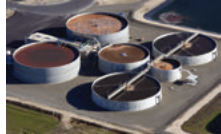
Anoxic & Nitrification Digester Tanks
