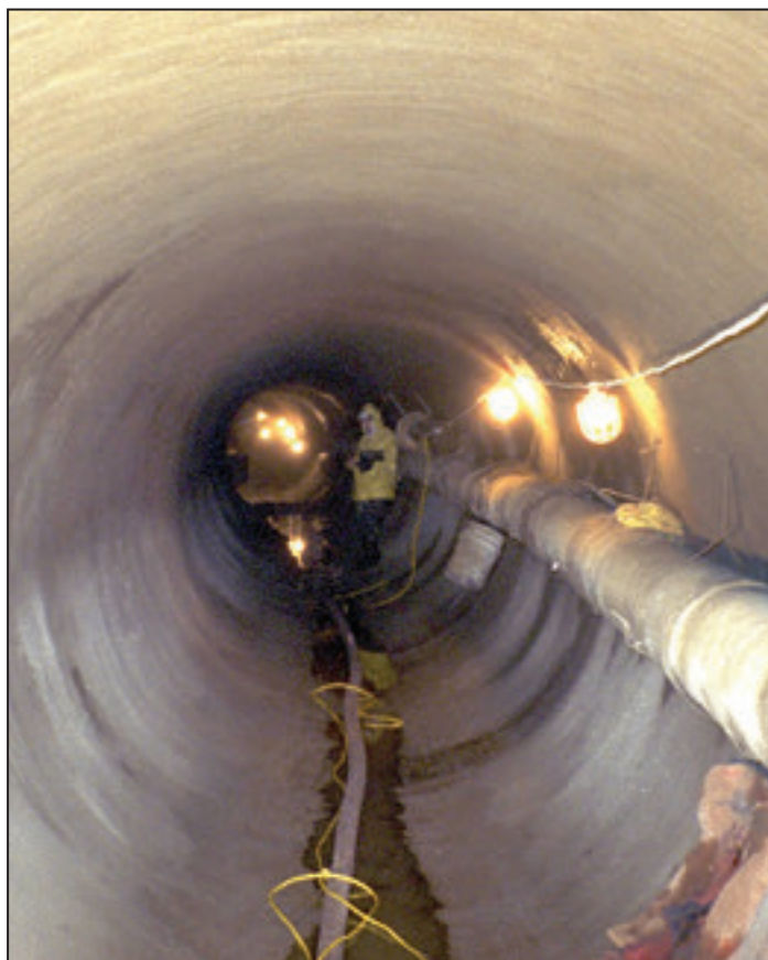
Performing structural rehabilitation of a large diameter sewer by gunite coating
