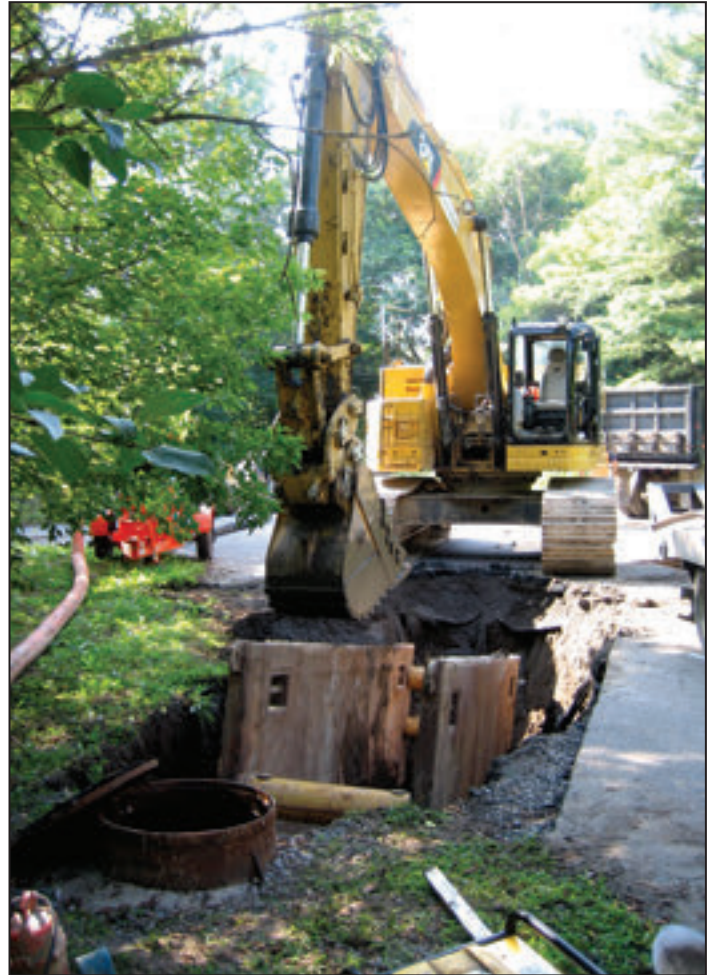
An open sewer repair in the Oneida County Sewer District
