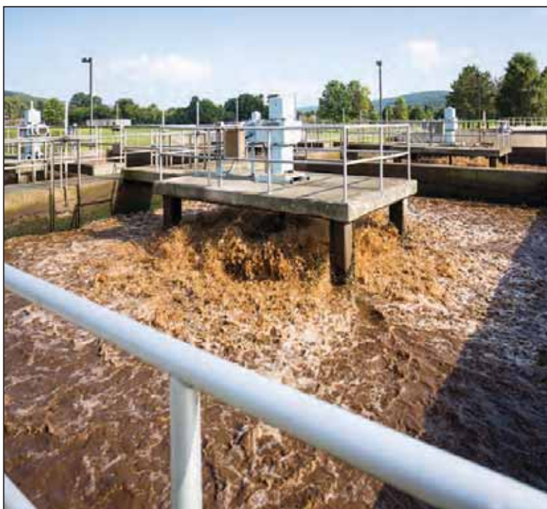
The existing surface aerators will be replaced with a more efficient aeration system.
