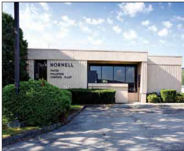
Hornell's Water Pollution Control Plant
