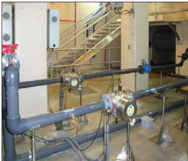
ETS-UV by Neptune Benson UV systems shown here used as part of AOP pilot study
