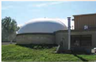
Digester Gas Holding Cover
