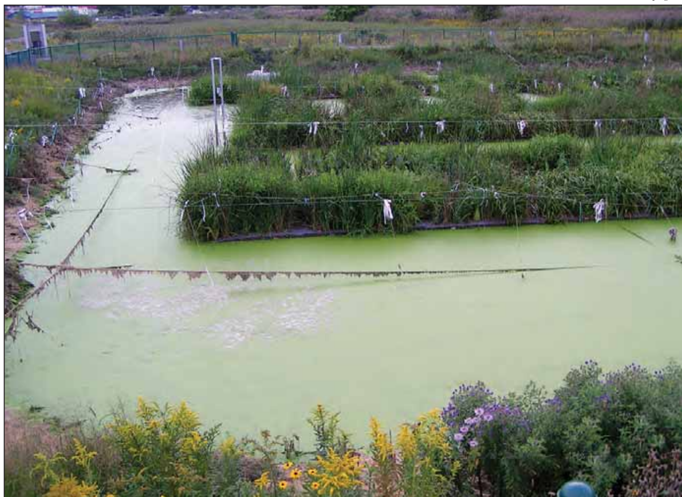
A constructed treatment wetland, such as this one, may use any combination of free water surface and submerged flow conditions to provide extended biological and physical treatment of contaminants of emerging concern. Vegetation provides treatment benefits, with secondary ecological benefits of habitat and aesthetic enhancement.
