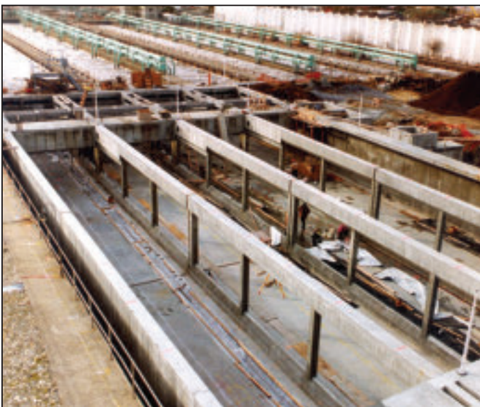
Figures 3A and 3B: Construction of the Phase 1 primary treatment upgrades, including the new primary splitter box (top) and the new primary settling tank (bottom)
