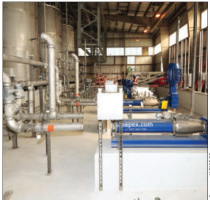
Figure 4. BNR upgrades at the 26th Ward WWTW include the construction of supplemental carbon addition facilities.
