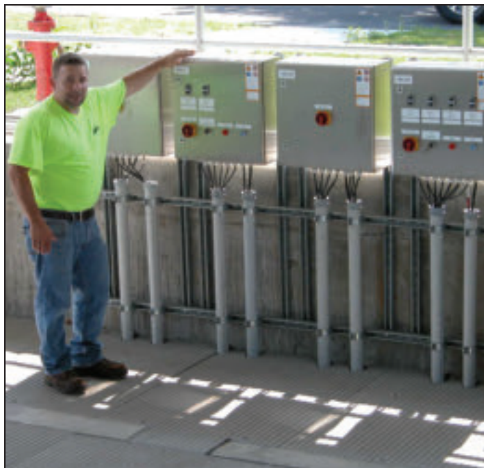
Vince Cordi stands next to control panels for the ultraviolet module lift and wipers at the South Plant.
