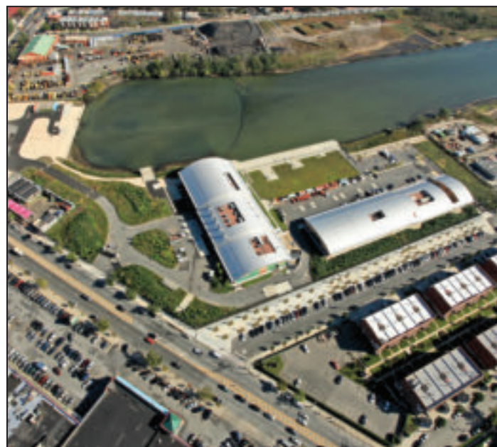
When the Paerdegat Basin CSO Facility, seen here, was placed into service in 2011, Paerdegat Basin greatly reduced CSO discharges to Jamaica Bay.
