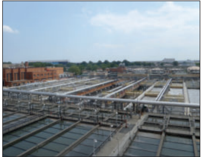
Figure 8. Jamaica WWTP aerial of completed aeration tanks
