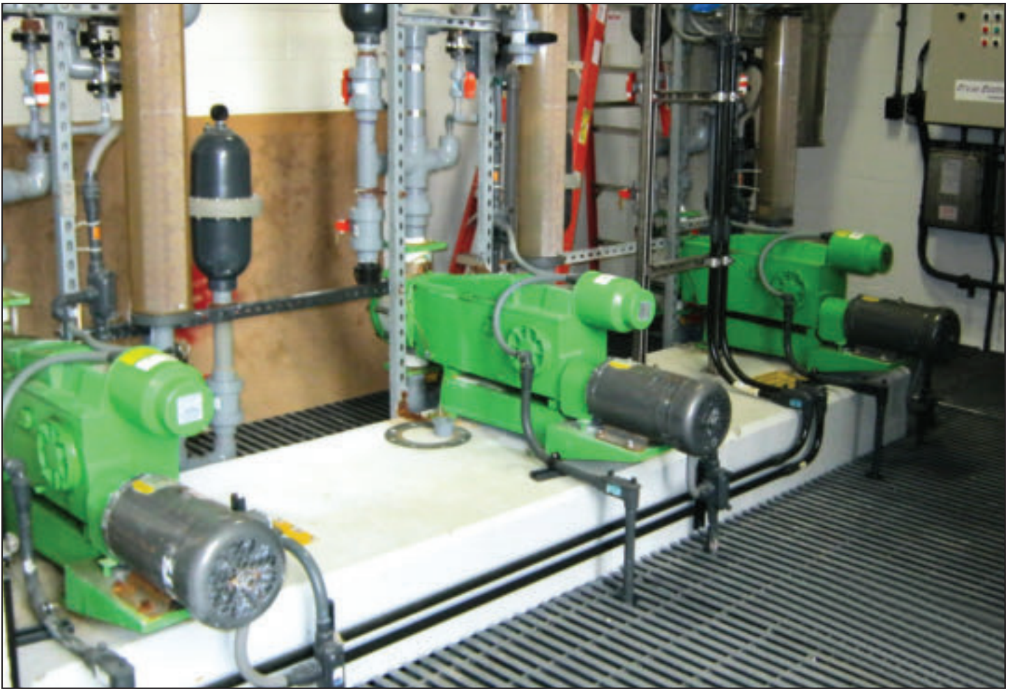
Figure 2. Existing hypochlorite metering pumps
