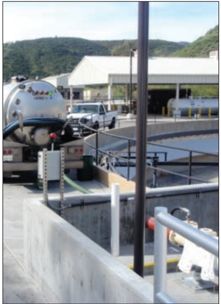
A FOG receiving station at a wastewater treatment plant
