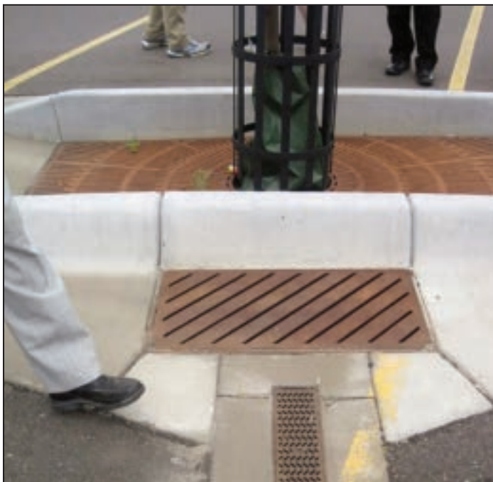
Stormwater tree trenches help channel excess water from the street through a trench or existing storm drainage, filtering and slowing the water along the way.
