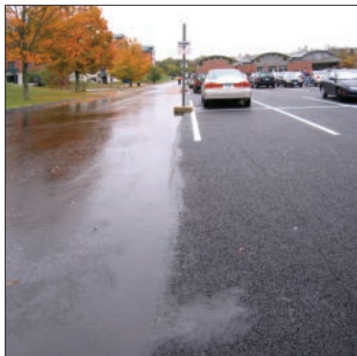
On the left is flooded, conventional street pavement; on the right is permeable street pavement that absorbs water to keep roads passable during heavy rains.
