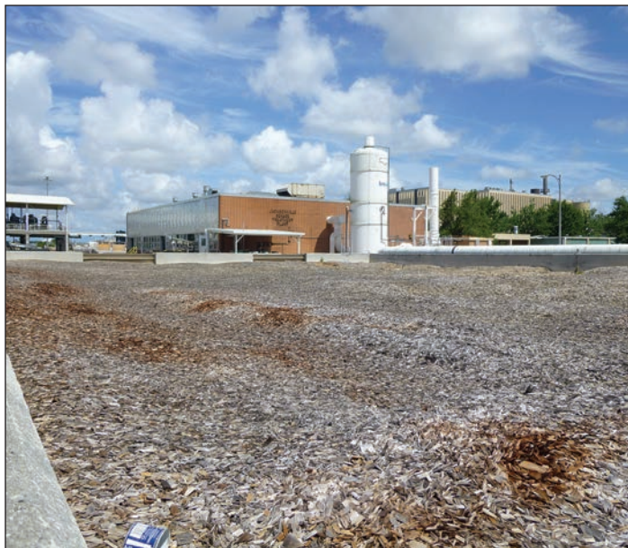
Figure 3. Biofilter treating approximately 7,000 cfm. Matt Johnson
