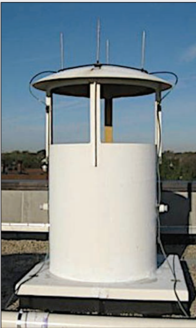
Figure 3. Odor control rain cap. Hazen and Sawyer
