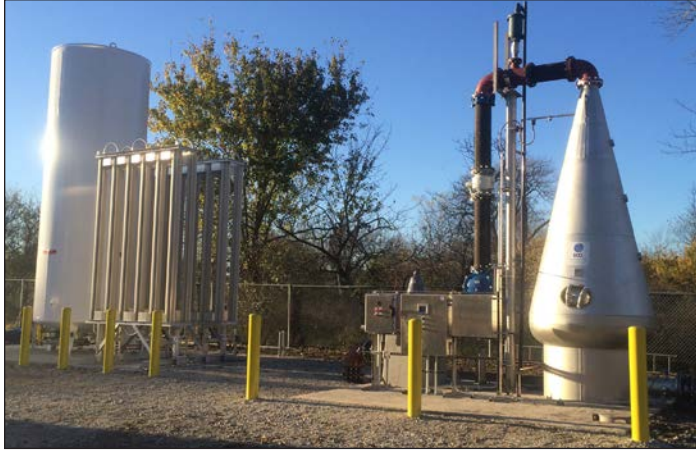
Oxygen dissolver used to control hydrogen sulfide.
