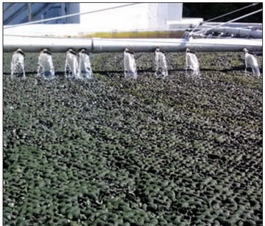
Algae is shown growing on a trickling filter which helps to remove phosphorus from waste naturally.
