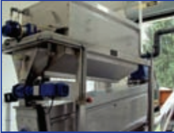
Groton NY WWTP Model 3012 DSP Screw Press
