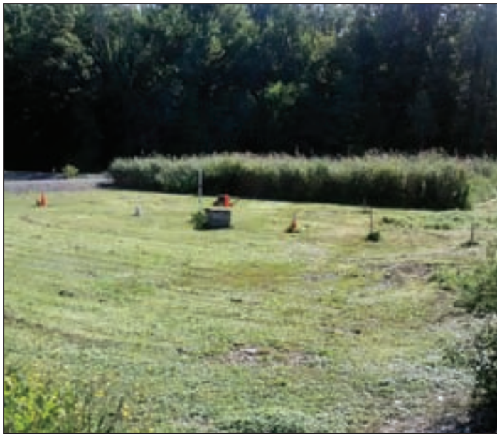
The facility's wetland with reed grass, filters contaminate compounds from wastewater.
