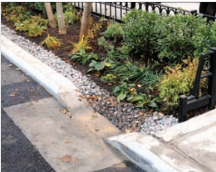
Above: Problems of clogging around the bioswales' curb plates resulted in modifications, such as depressed curbs seen in the lower photo.
