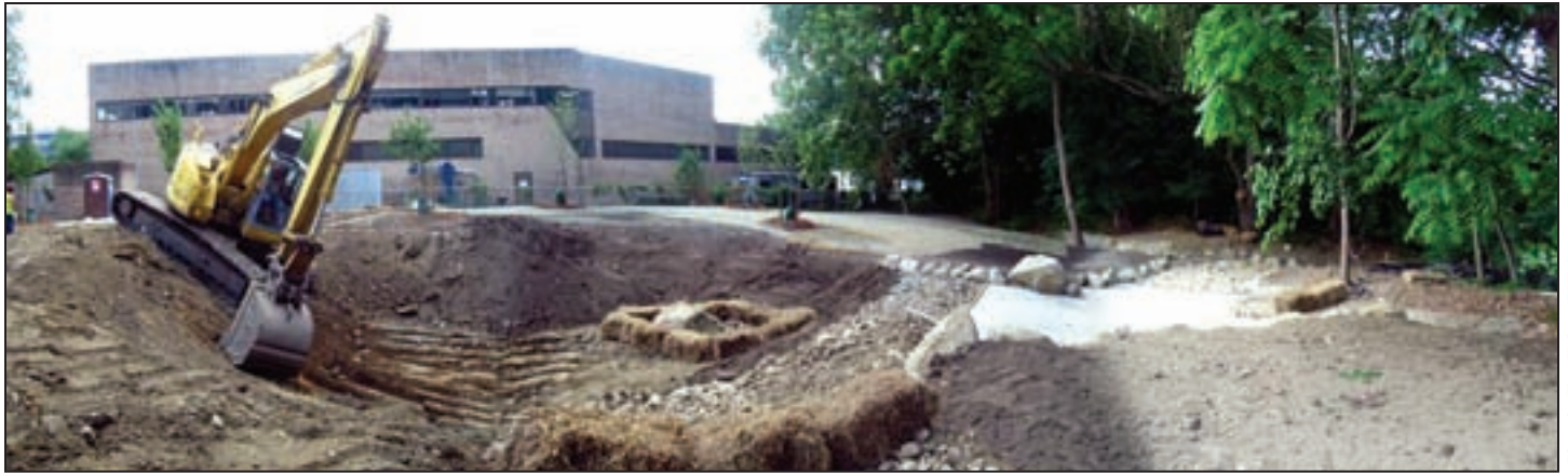
Rain garden during construction. Straw bales surround diffusion well during this phase and protect voids from clogging with sediment (Site No. 5).
