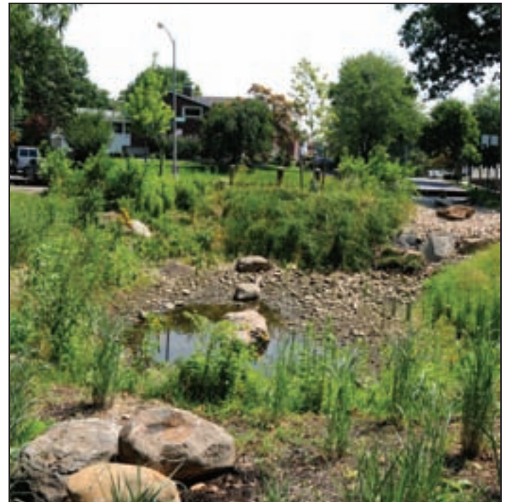
The completed rain garden intercepts stormwater flows from the surrounding streets, and promotes infiltration (Site 5).
