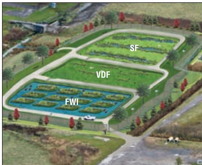
Figure 1. The Harbor Brook Constructed Wetlands Pilot Treatment System incorporates three types of wetland cells – from bottom to top: Floating Wetland Island (FWI), Vertical Down Flow (VDF) and Surface Flow (SF).
