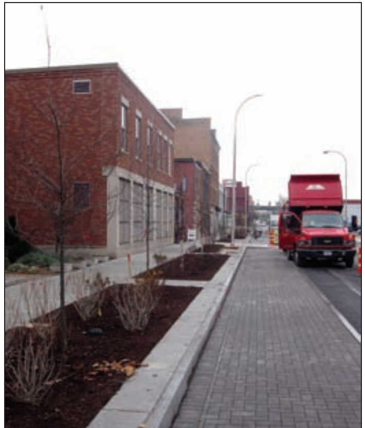
The scope of the Water Street Gateway project will incorporate streetscape detail with enhanced tree plantings in the right-of-way; installation of porous pavers in parking lanes; use of infiltration trenches and planters; and additional landscaping features throughout the footprint of the block.
