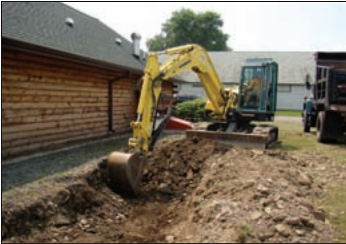
Excavation for a bioretention demonstration project at the Chemung County Fairgrounds – a green effort by the Chemung County Stormwater Coalition to help filter pollutants and manage stormwater runoff at the site. Equipment used was donated by the County Soil and Water Conservation District, and plant and soil materials to complete the project (shown in second photo), were donated by Natural Resource Conservation Services.
