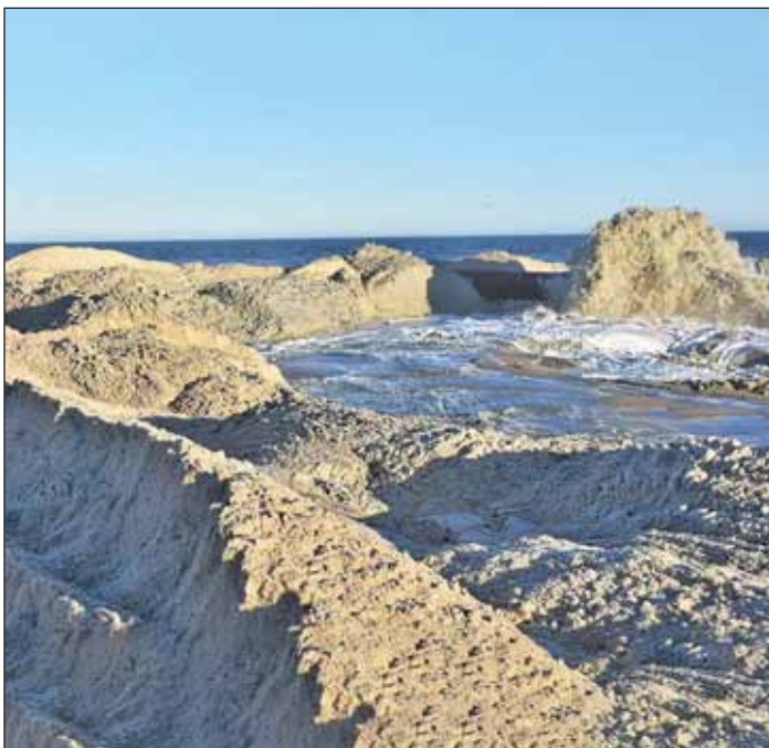
Photos show sand being pumped through pipelines onto Gilgo Beach, one of several beaches receiving sand replenishment with The Fire Island Inlet to Montauk Point, New York, Coastal Storm Risk Management Project.
