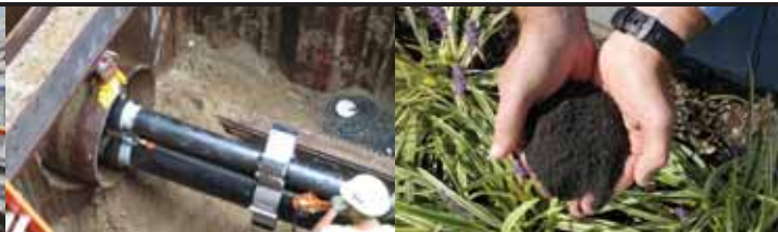
Ronkonkoma Hub Pump Station
