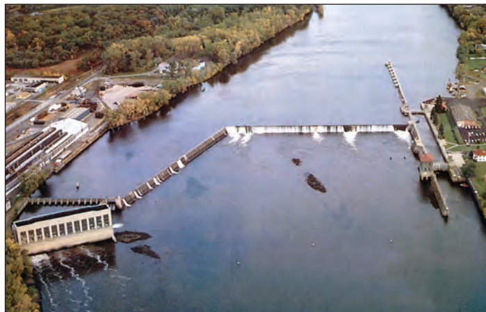
Aerial view of the Troy Lock and Dam in Troy, N.Y.
