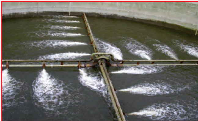
JET MIXING IN EQUALIZATION TANKS
