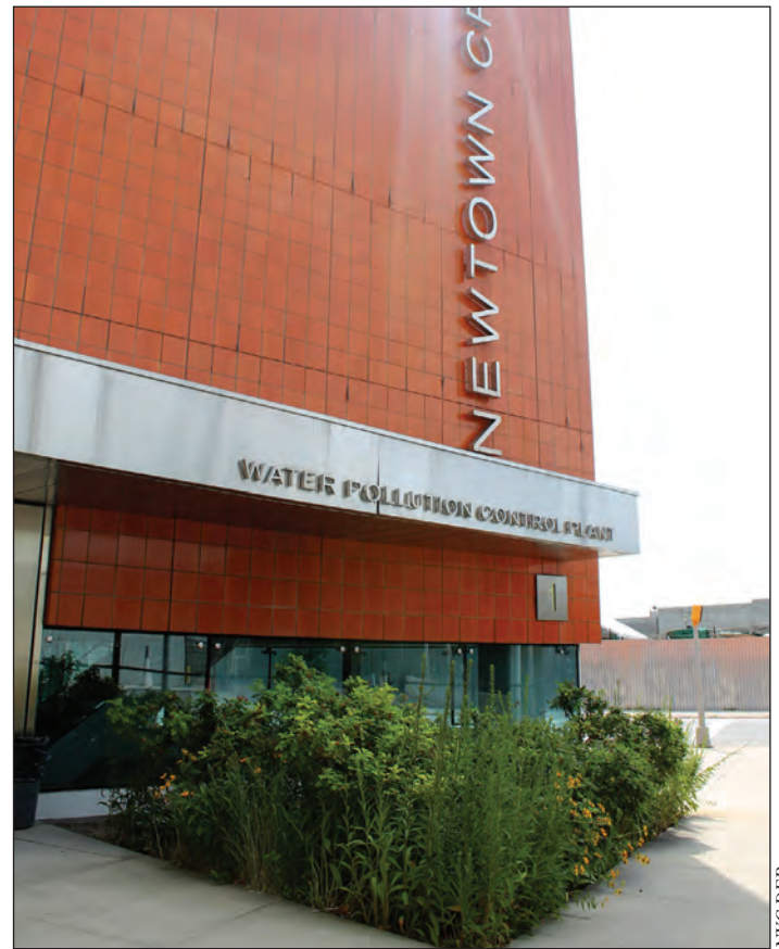
A distinct feature of the Newtown Creek Wastewater Treatment Plant is the bright orange facade of the Visitor Center along Greenpoint Avenue.
