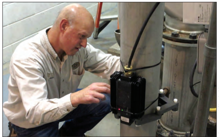
Douglas Miller installing Unit 2 on centrifuge feed pipe
