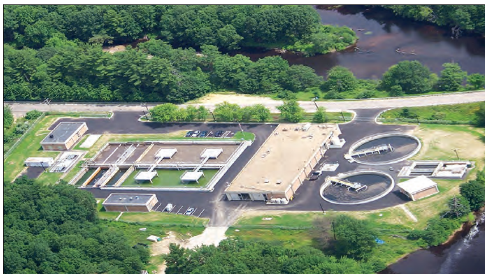
Aerial view of Somersworth Water Resources plant, Somersworth, N.H.
