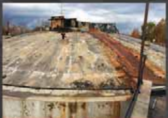
Digester Roof Replacement
