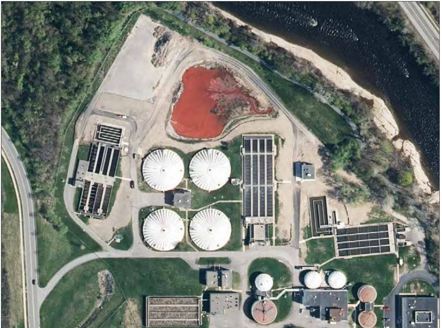
Aerial image of the City of Watertown Pollution Control Facility.
