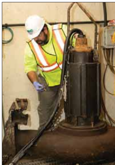
Photograph 2. Collections Sewage Treatment Worker checking a submersible pump before installation.
