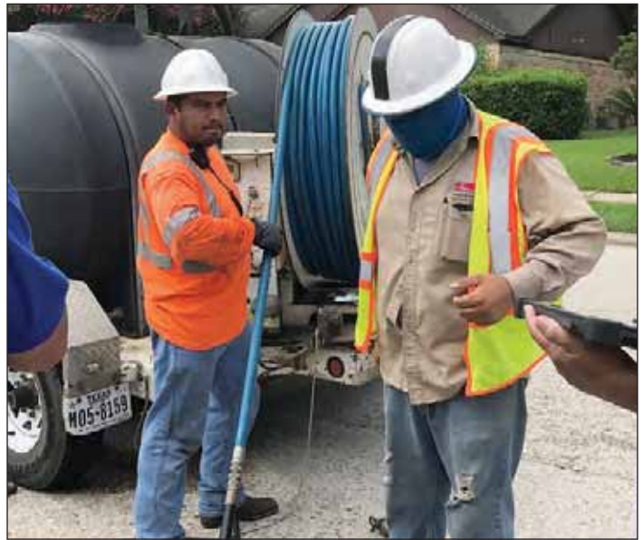
Photograph 1. Workers cleaning a collection system.
