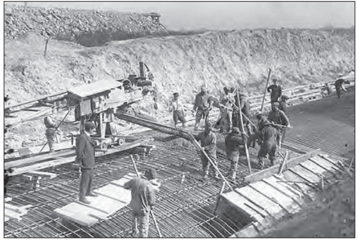
Pouring the concrete on the roof of the drain.
