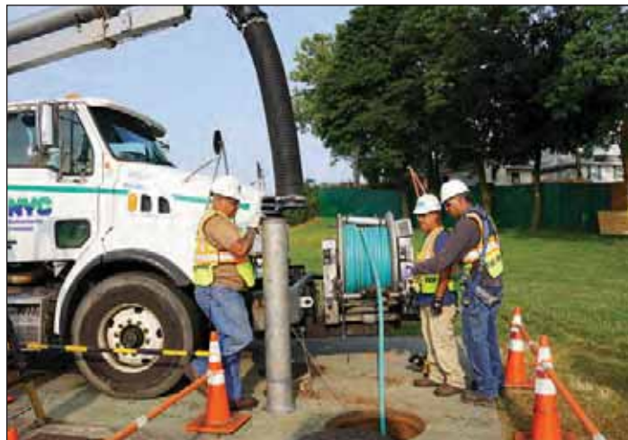
Photograph 5. DEP Collections crew "vactoring" a chamber.
