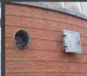
Wall Access Upgrade
