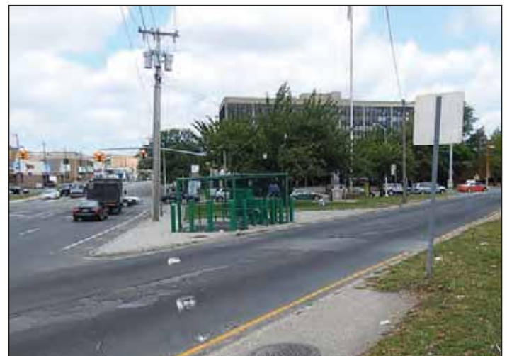
Photograph 1. The southerly side of the Weekes Park Pump Station site, Aug. 19, 2014, pre-design, viewed looking north. The flagpole, monument and original hydrant location are visible. Access to the original below-grade pump station is located within the green fence.
