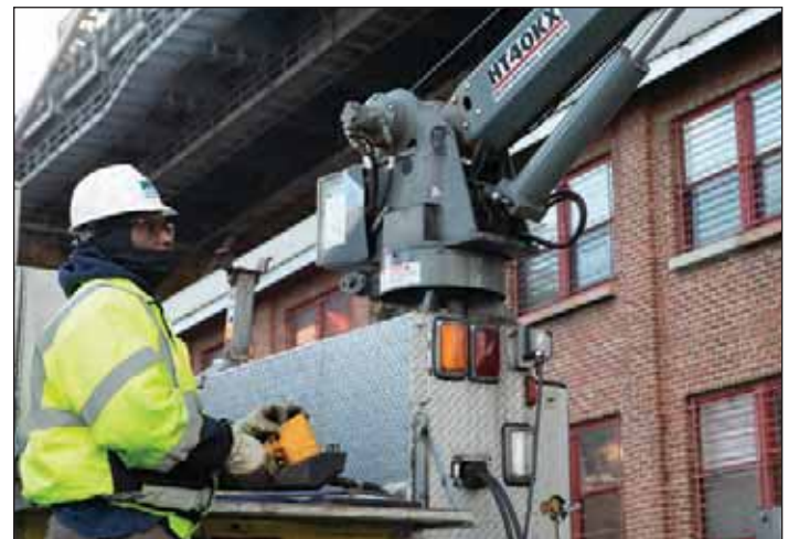
Photograph 1. Collections Sewage Treatment Worker operating truck-mounted crane to exercise a tide gate.
