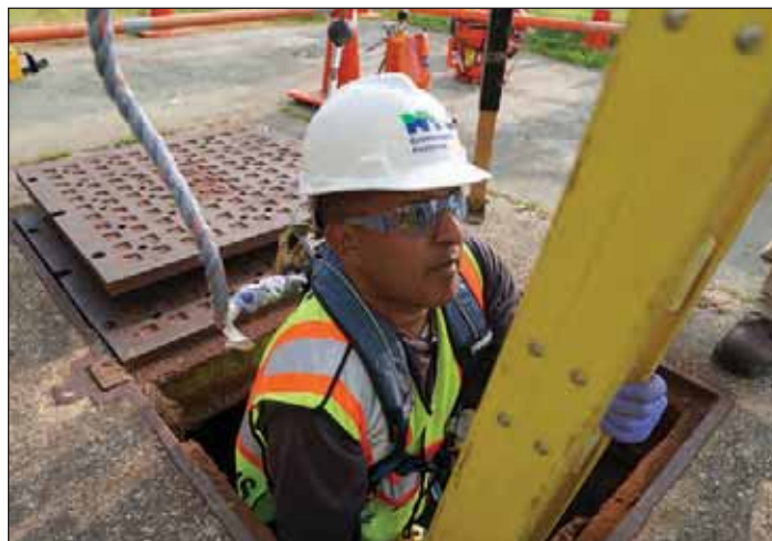
Photograph 4. Senior Sewage Treatment Worker Victor Basdeo inspecting a regulator in the Bronx.
