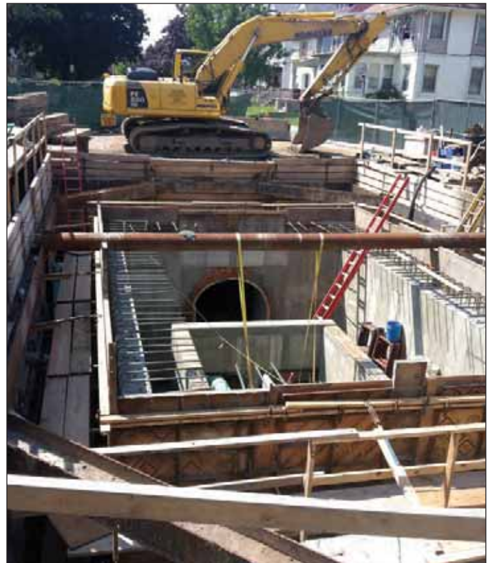
Figure 2. Construction of the Bird RTC chamber.
