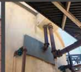
New Pipe Penetrations
