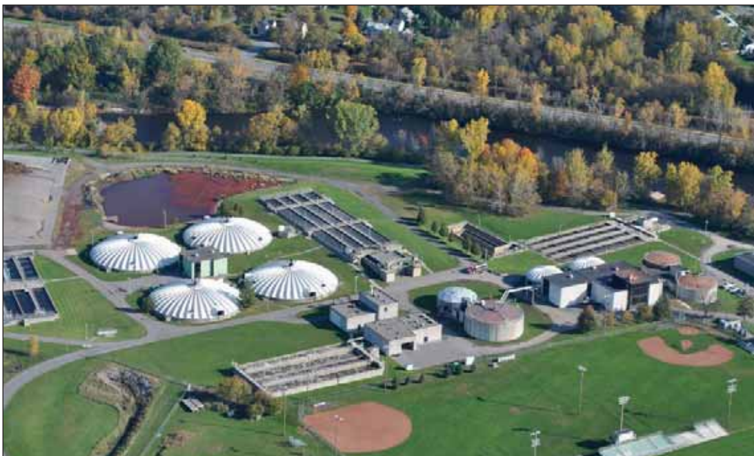
Aerial view of the City of Watertown Pollution Control Facility.
