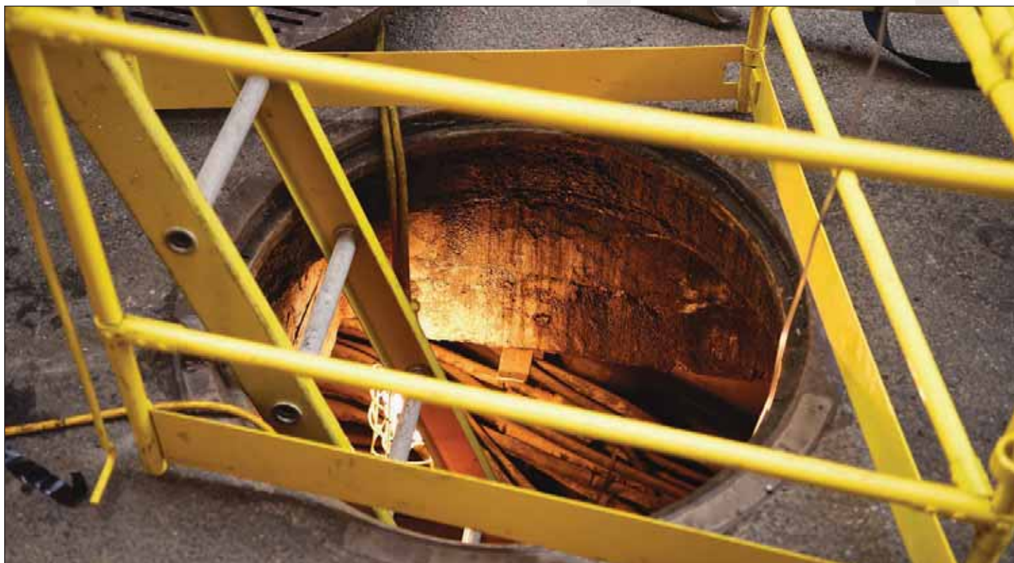
Care must be taken to ensure safety when using ladders. Pay attention to the angle of the ladder, the extension above the landing, and the stability of the base.
