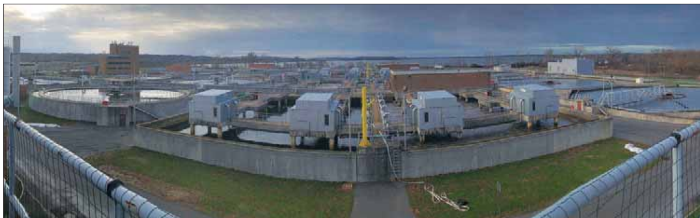
Panoramic view of a water resource recovery facility.
