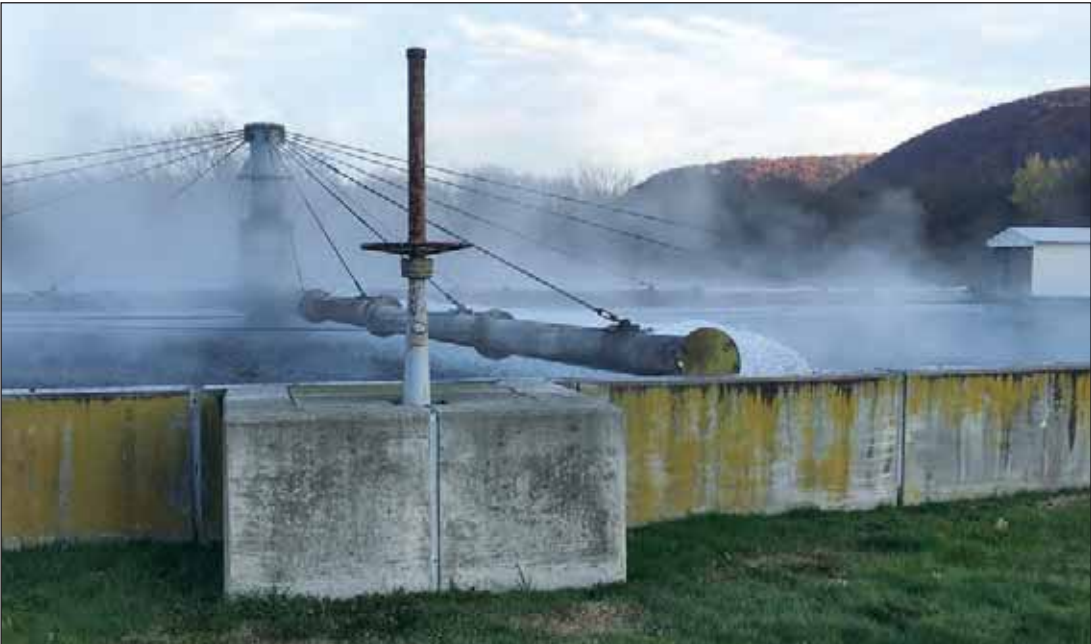
Photograph 2. The Lake Street Plant’s trickling filters will be decommissioned.
