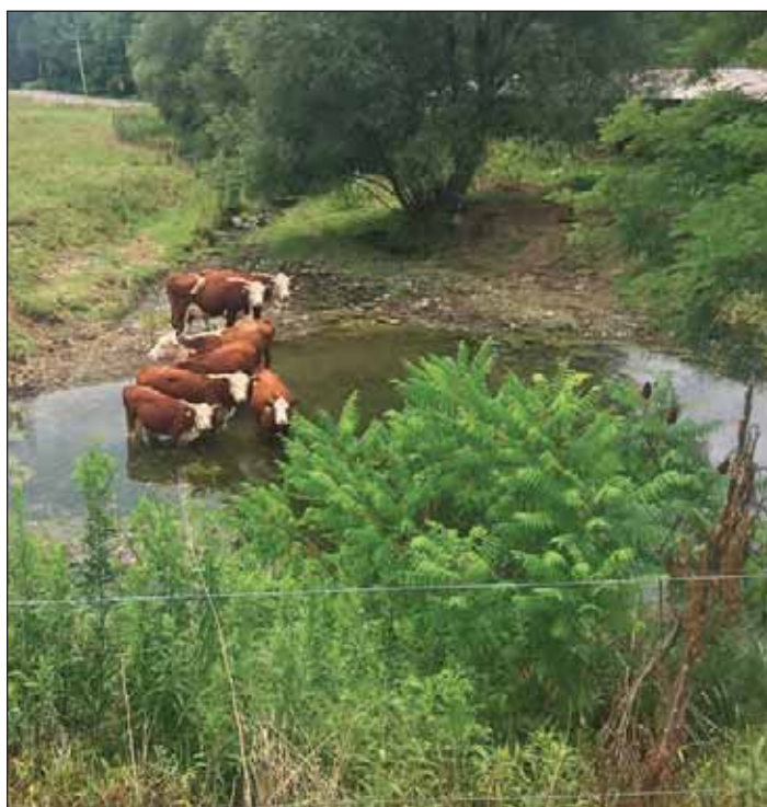
BEFORE: View from the culvert outlet, looking downstream. Cows were free to wade in the stream, contributing to erosion and nutrient release.
