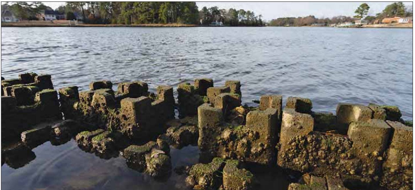
Indian River in Chesapeake, Virginia. A shoreline restoration project is seen near homes on the Indian River Dec. 16, 2019. In 2018, resident Rogard Ross worked with the Elizabeth River Project and secured permission from his condo association to construct a 550-foot living shoreline in his neighborhood. In addition, 200 volunteers helped install 800 oyster castles and 5,000 native plants, including saltmarsh cordgrass and saltmeadow hay. The project helps protect the residents’ shoreline from erosion. Will Parson/Chesapeake Bay Program
