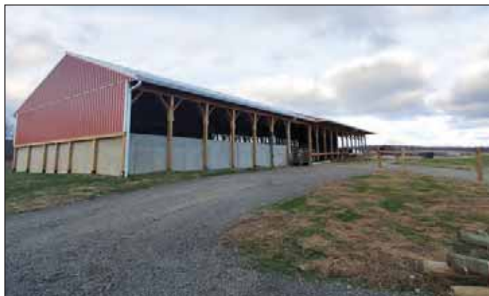
Photograph 1. The finished covered barnyard and manure stacking pad. Tioga County SWCD
