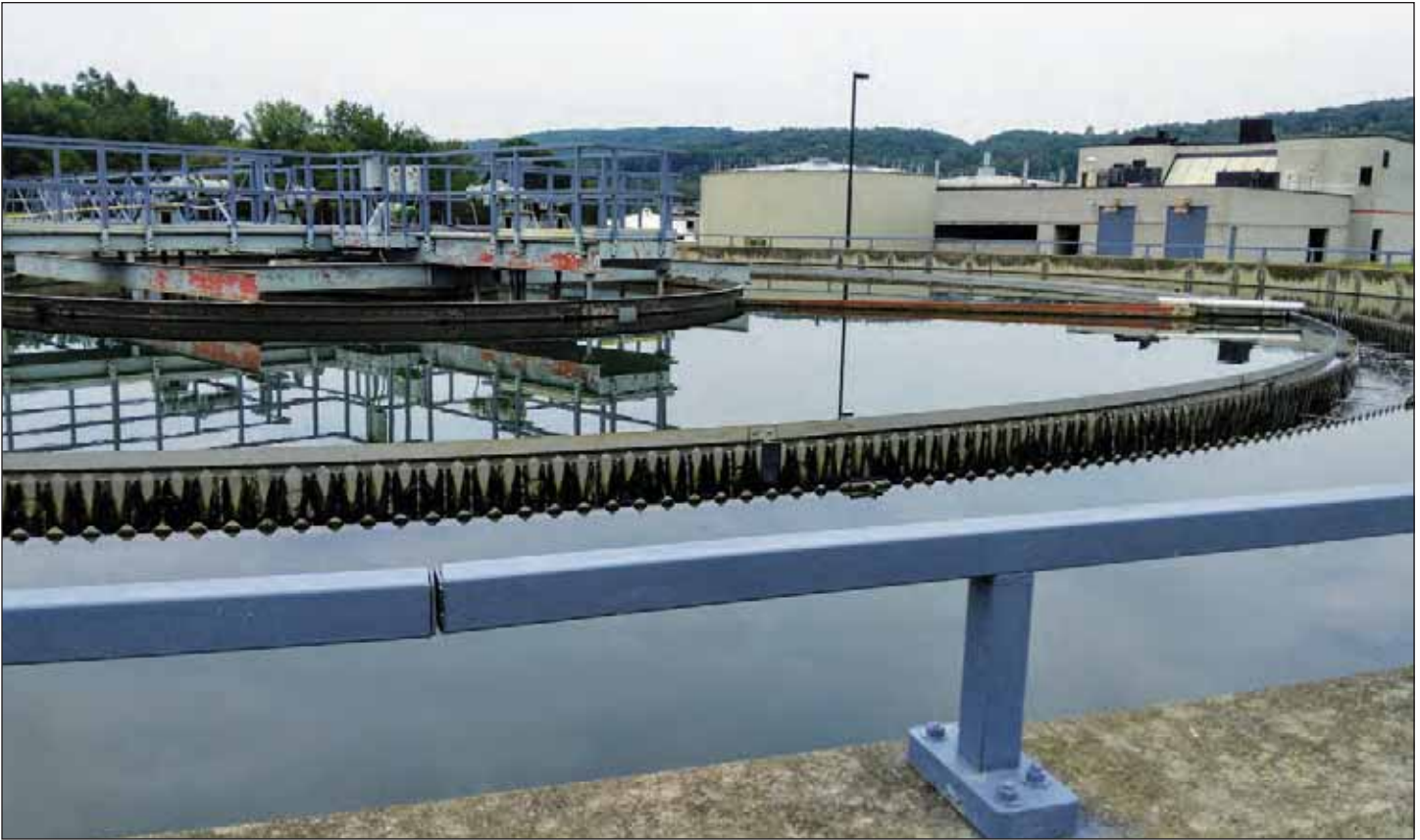
Photograph 1. The existing Milton Street Plant, with clarifiers in the foreground and the solids handling buildings behind. The steep hills that form the Chemung River valley are visible in the background.
