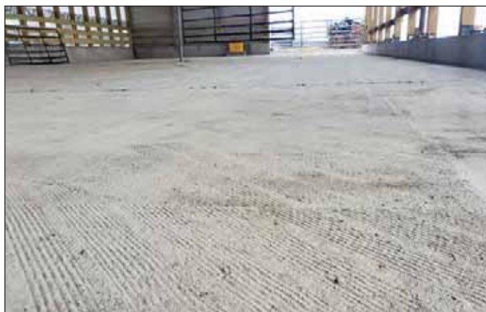
Photograph 3. Traction milling technique on the concrete floor. Tioga County SWCD
