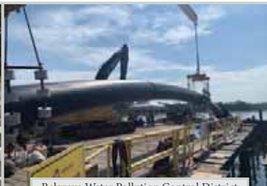
Belgrave Water Pollution Control District
