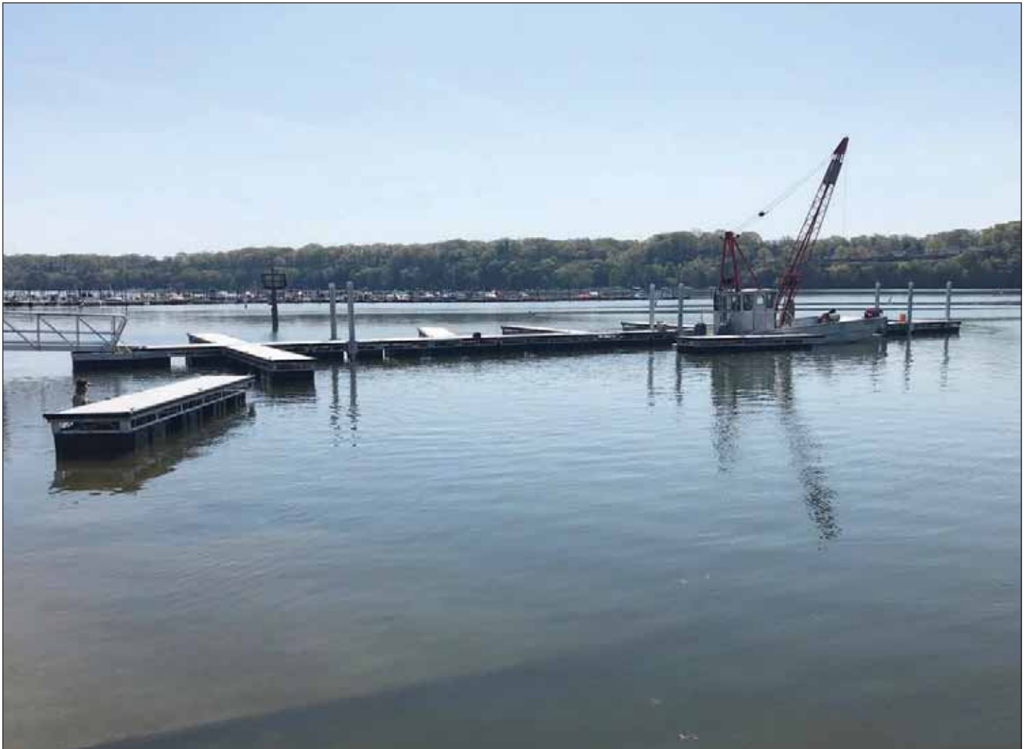
Photo 3. Installation of transient dock systems for boater parking to support local businesses – capacity of 24 boats.
