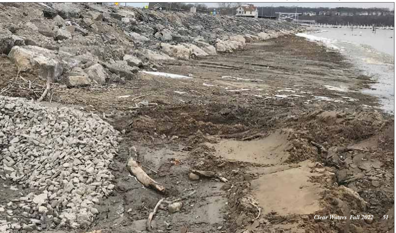
Photo 6. New stormwater outfall and pump station discharge Ramboll, 2020
