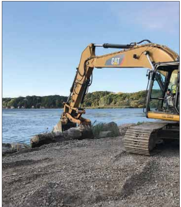
Photo 5. Revetment installation to provide long-term flood protection. Ramboll, 2020
