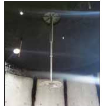
Energy efficient digester mixer at the IAWWTF. Jacob Yousey, Barton and Loguidice
