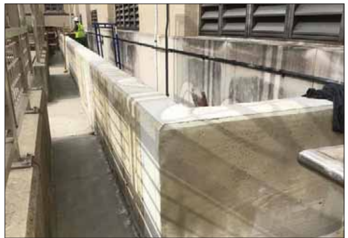
Typical flood wall to protect critical infrastructure. AECOM
