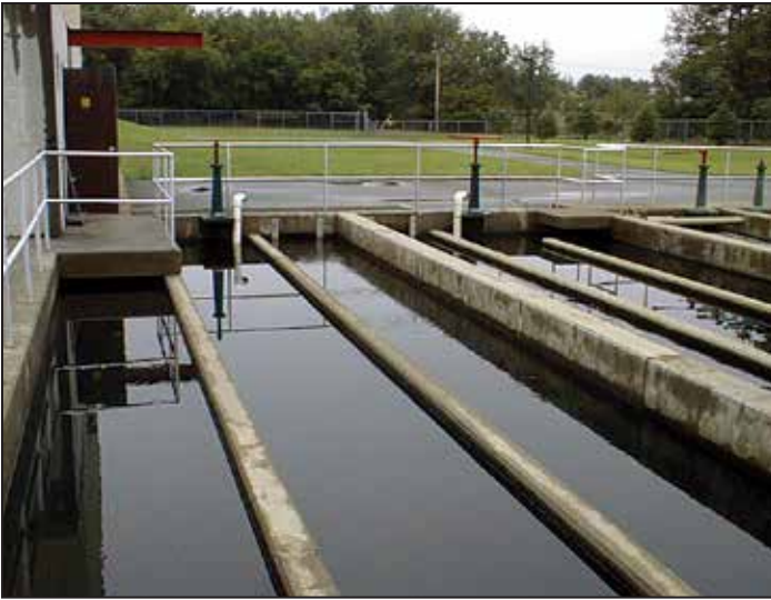
A chlorine tank that is well monitored
