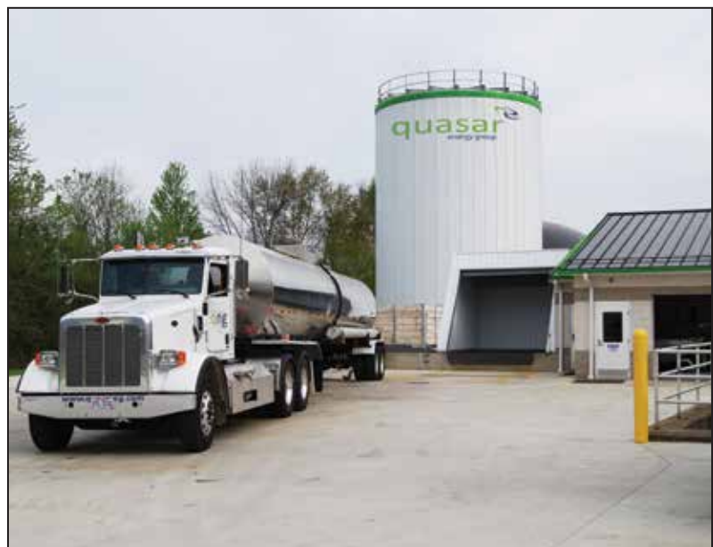
A biomass equalization tank is used to mix the treatment plant solids with other substrates, such as food wastes, prior to loading into the digesters.
