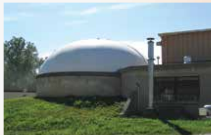
Digester Gas Holding Cover
