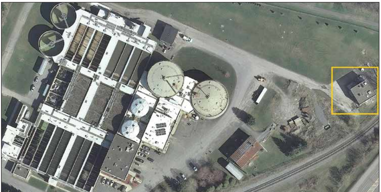
The Ithaca Area Wastewater Treatment Facility where an enhanced primary treatment technology was piloted through a NYSERDA grant. The boxed building shows where the EPT pilot was placed for testing.
