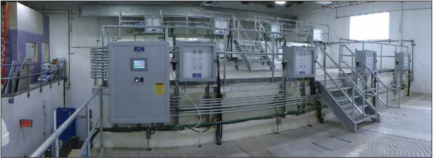
The two-stage filter system consists of four filter trains, each with two filter units. Each filter is covered by a solid-surface aluminum deck panel. The influent channel distributes water pumped from Well 5 to the first stage filters (background) which include 80 inches of filter sand. Water then flows by gravity to the second stage filters that have 40 inches of sand. Each filter has a dedicated air panel controlling the backwash processes. A central control panel (left) manages and reports on filter operation and backwash activities.
