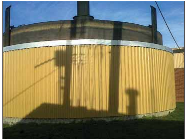
A floating digester cover that provides a small amount of biogas storage volume
