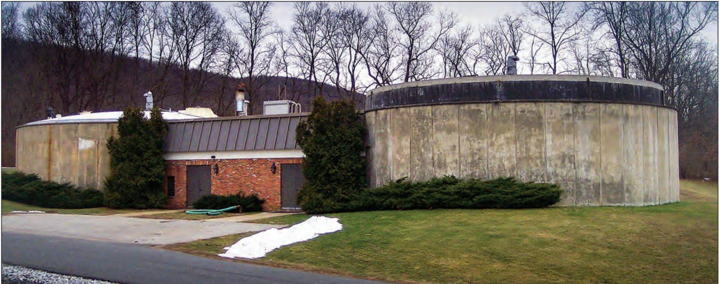
Typical primary and secondary anaerobic digesters
