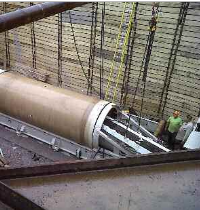
Installation of 84-inch diameter HOBAS piping by trenchless/pipe jacking method. Shown is the initial setup of the open-faced tunnel boring machine (TBM) and first pipe section for a 300-foot tunnel run.
