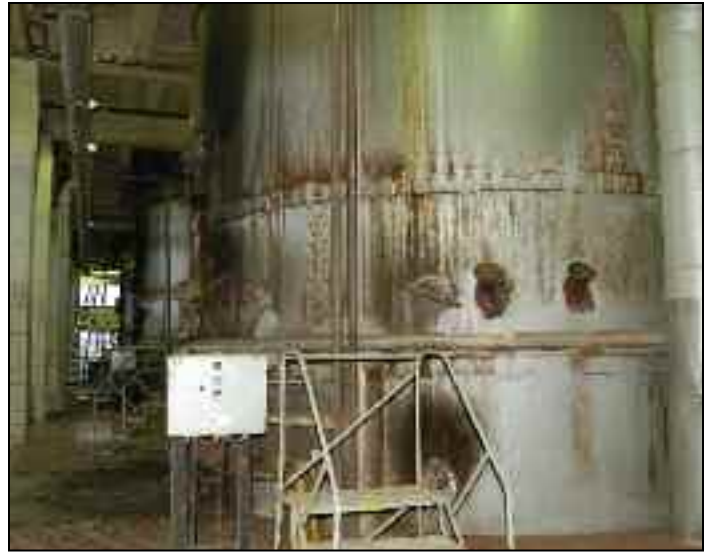
Photo by Buffalo Sewer Authority
