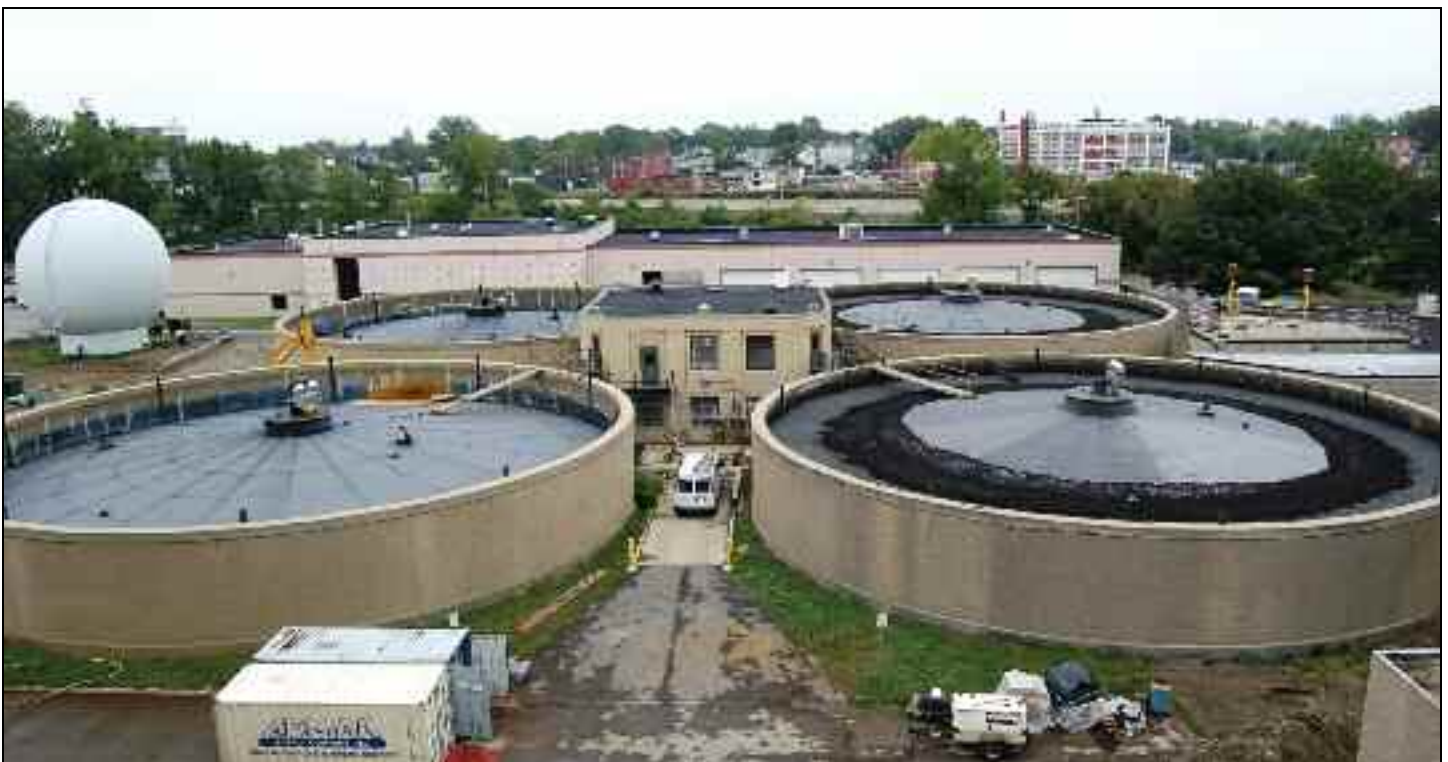
Photo by Buffalo Sewer Authority
