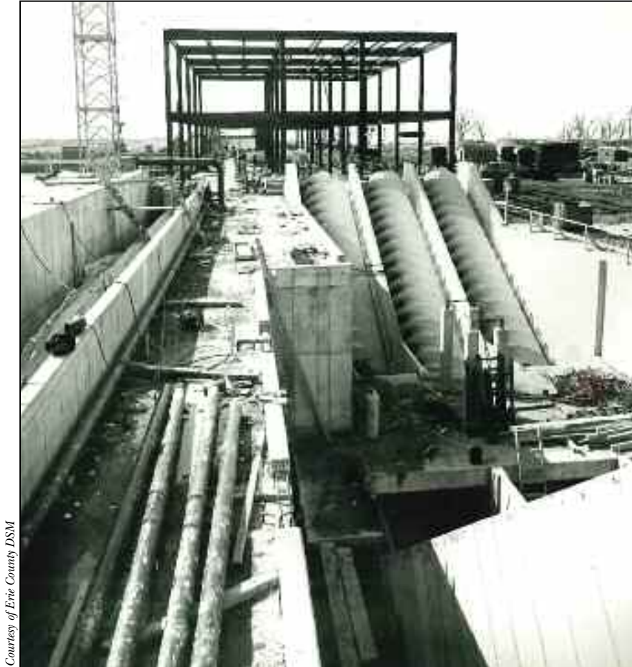
Screw pumps at the Southtowns Advanced Wastewater Treatment Facility during construction in 1979
