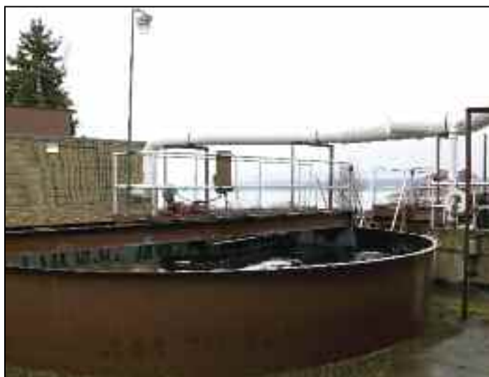
A secondary clarifier tank next to the rotating biological contactor building at Chautauqua Utility District's wastewater treatment plant, adjacent to Lake Chautauqua
