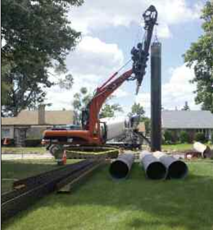
The removal of a 30-inch diameter shaft casing used for installation of the 40-foot long soldier piles for an overflow chamber, a project component, within a residential neighborhood.
