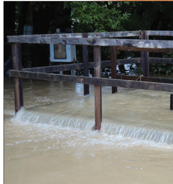
Flooding of the sampling manhole for influent flows
