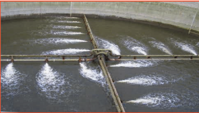
JET MIXING IN EQUALIZATION TANKS
