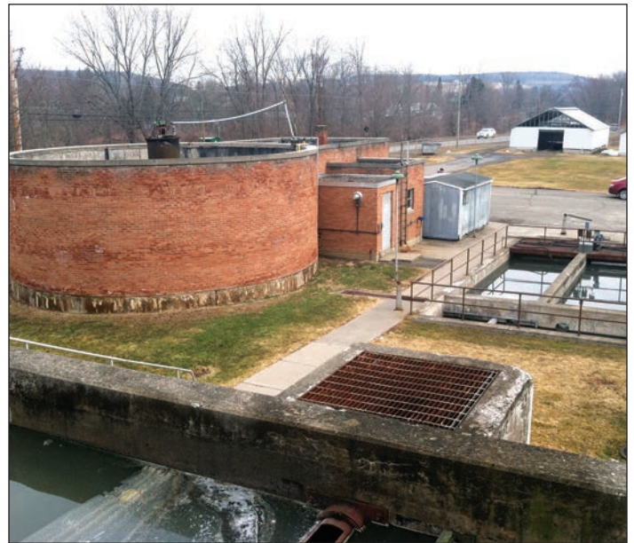
Existing facility shown here contains the control building, aerobic digester and clarifier.
