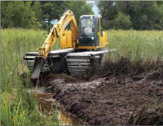
Figure 3. U.S. Fish and Wildlife Service operates an aquatic excavator with cutter head to create channels; side-casted material has been shown to contain viable native plant propagules that germinate following re-exposure.
