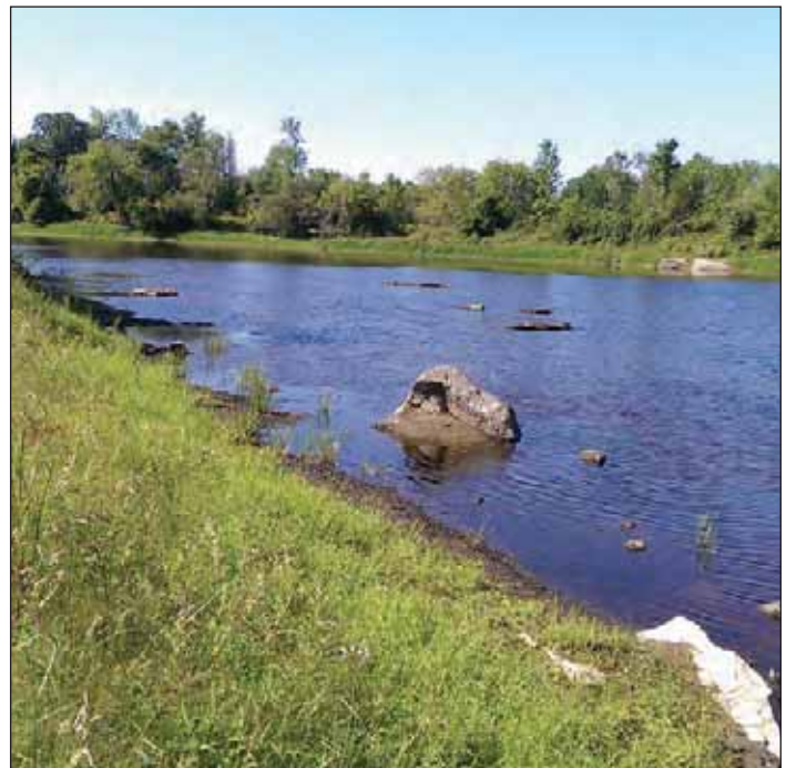
The banks within the impoundment, exposed after drawdown, were revegetated to stabilize the sediments left behind. Tony David, SRMT
