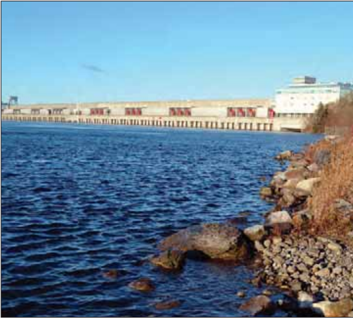
Moses-Saunders Dam located near Cornwall, Ontario and Massena, New York, is the main control structure on the St. Lawrence River used to regulate outflows from Lake Ontario. Environment Canada
