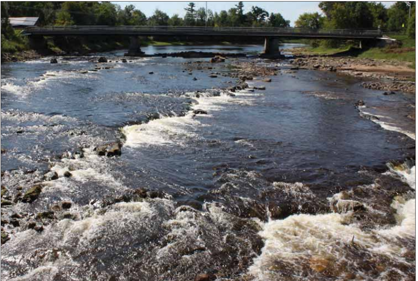
The impoundment after dewatering. The limited volume of sediments was naturally distributed. The flow and sound of cascading water was restored.
