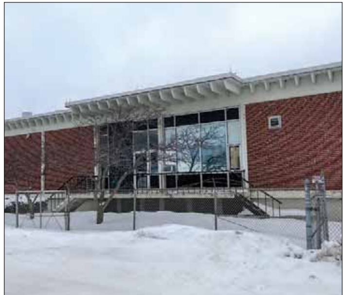
The spatial use within the WRRF Control Building will be reconfigured as part of the overall project. Charles Prior
