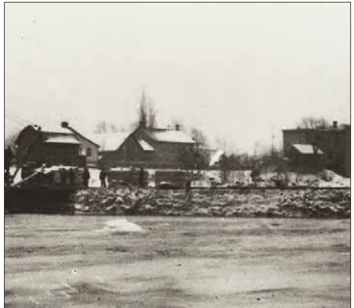
The former timber dam and primitive crib dam at Hogansburg, New York. This dam was eventually breached by ice floes in 1905 during the spring freshet.
