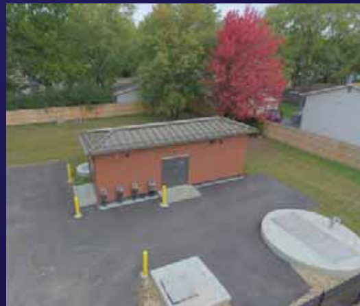
Prefabricated Housed Pumping & Equipment Systems
