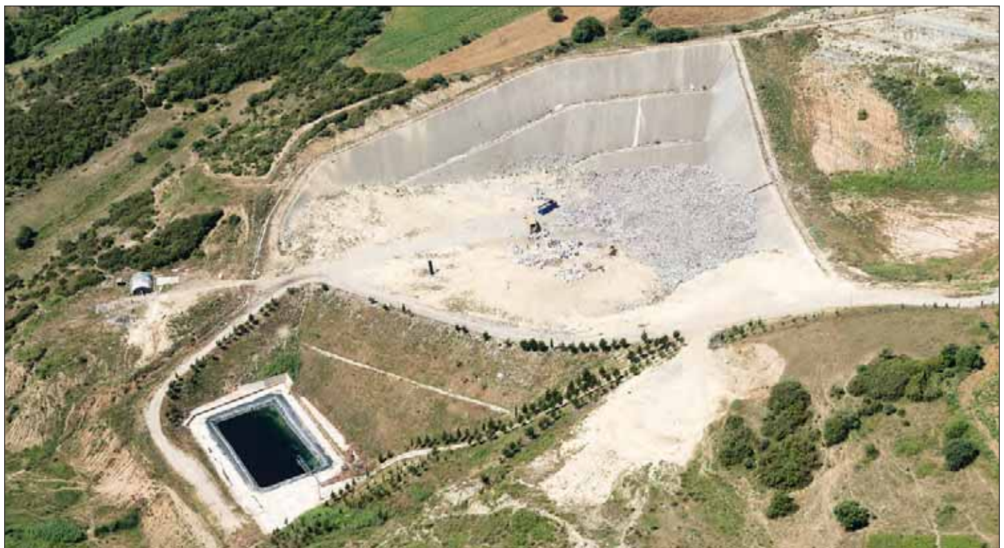
Modern landfill construction design includes leachate capture systems, which protect local groundwater.
