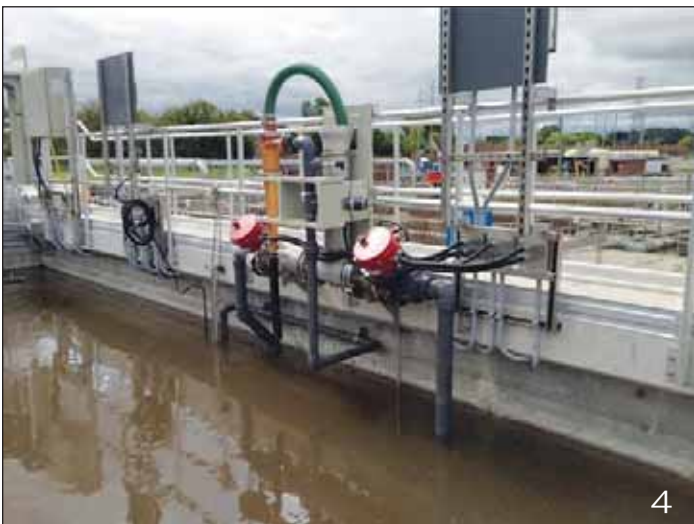
Clockwise: Photograph 1. Sidestream hydrocyclones at AlexRenew Water Resource Recovery Facility, Alexandria, Virginia; Photograph 2. Anammox granules at AlexRenew Water Resource Recovery Facility; Photograph 3. Sidestream reactor at Guelph Wastewater Treatment Plant; Photograph 4. Sidestream hydrocyclones at Guelph Wastewater Treatment Plant, Guelph, Ontario, Canada.
