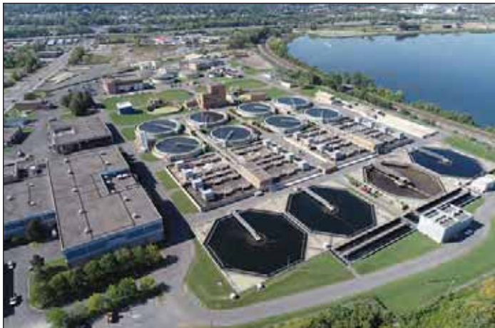
Photograph 1. The Metropolitan Syracuse Wastewater Treatment Plant (Metro). Credit: OCDWEP
