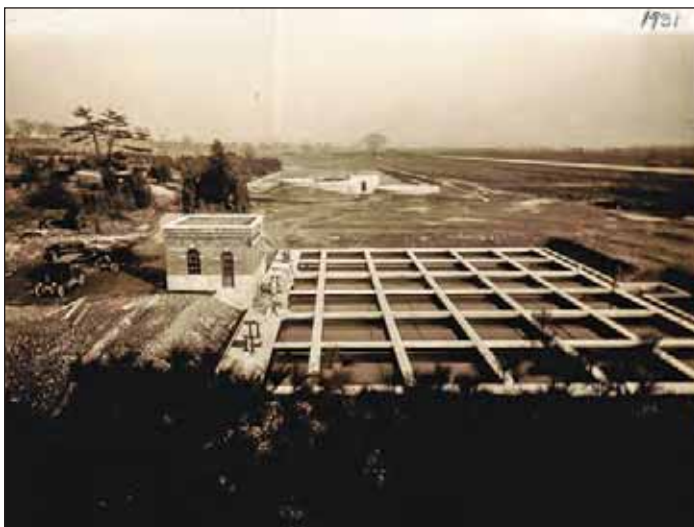
Photograph 1. A view of the original plant with discharge going directly to the Barge Canal seen on the right side of the photo. Credit: Hendricks, 1937
