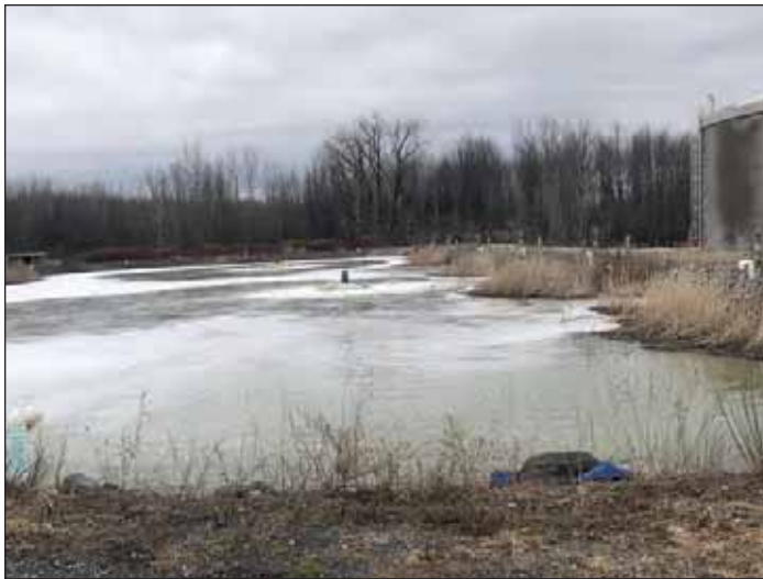
Photograph 6. The new storage tanks are adjacent to the discharging lagoon at the airport. Credit: OCDWEP
