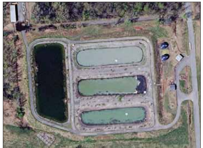
Photograph 2. Aerial image of the Syracuse Hancock International Airport original treatment lagoons.
