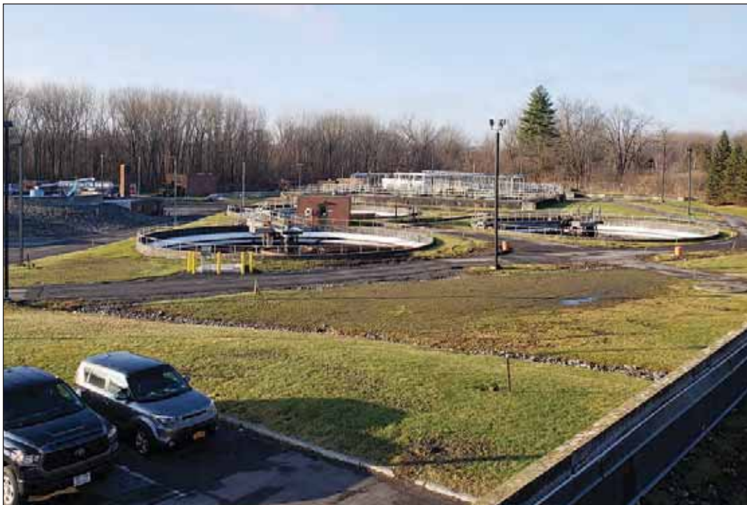
Photograph 3. Secondary process with aeration upgrade from mechanical aeration to fine bubble diffuser shown in the middle of the far back.
