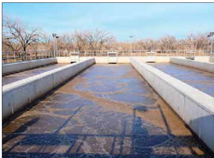
Photograph 1. Treatment tanks at the Havre Wastewater Treatment Facility, Jan. 24, 2020.
