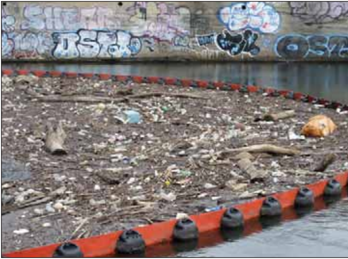
Floatables trash boom installed at Concrete Plant Park (Bronx, NY) in 2014
