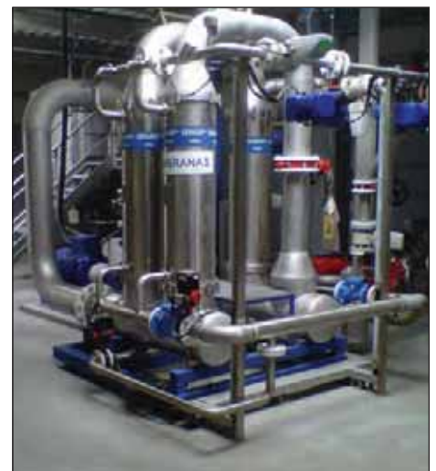
Figure 1. The biological reactor with the mechanical HPO injection aerator tank (left), equalization tank (center) and the membrane system (right)
