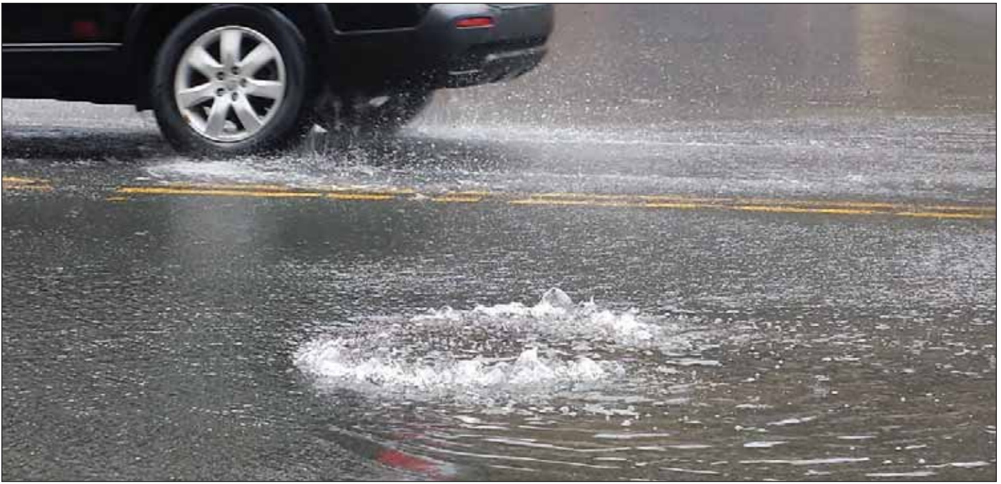
This CSO discharge to the Hudson River needs to be reported.
