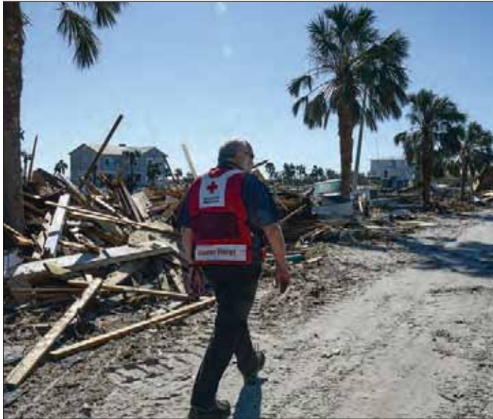
Hurricane Michael, October 13, 2018, Mexico Beach, Florida. Hurricane Michael inflicted a monstrous amount of damage to this beach-side community as it slammed into the Florida Panhandle with almost 150 mile per hour winds. Boats were tumbled every which way on the shore along harbor areas and even well inland. Homes were blown completely off foundations and tossed many yards away, and in many cases, homes were reduced to construction rubble. Almost every building suffered severe damage. The damage was so extensive the curiosity was the very few homes or businesses that did not have observable severe damage instead of the norm of devastation. Daniel Cima/American Red Cross
