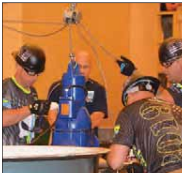
Rockaway Sludge Hustlers ably handle performing service on a KSB submersible pump.
