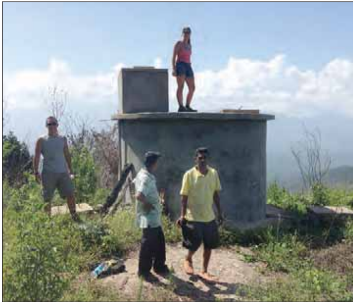
Taylor standing on a water storage tank in Buena Vista, Honduras. SUNY-ESF's EWB college student chapter partnered with the community to design and build a gravity-fed water supply system. Theodore Endreny
