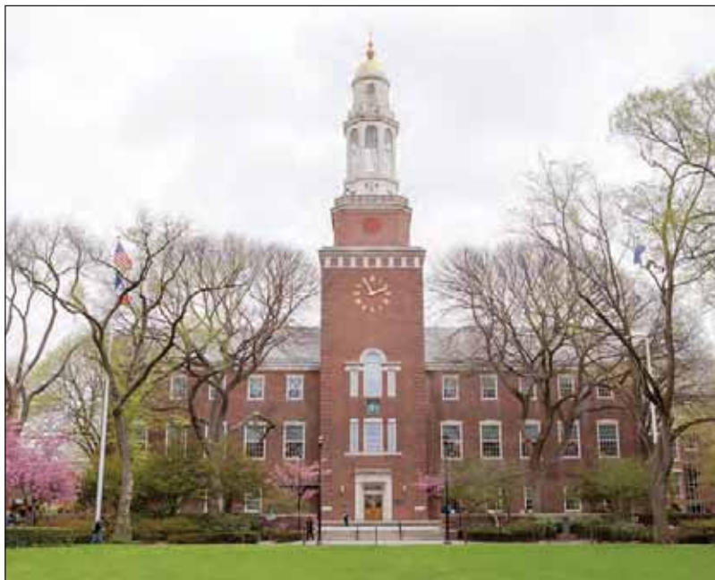
The Brooklyn College Library with its clock tower is an iconic landmark in the borough.
