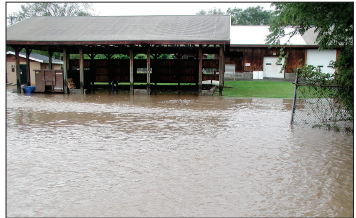
Above: Flooded drying beds at a wastewater treatment plant
