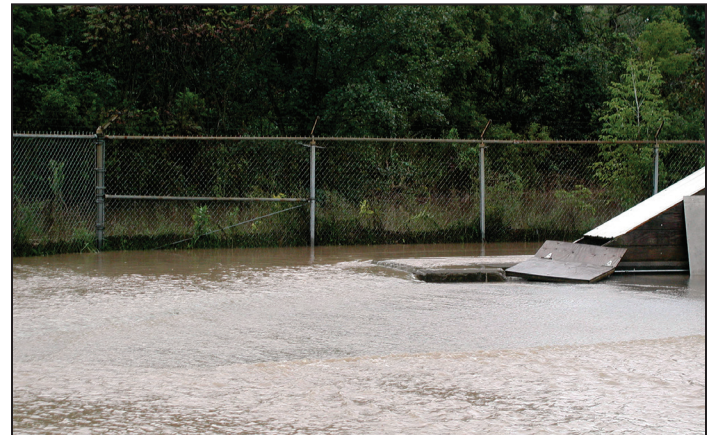
Below: Influent channel flooding
