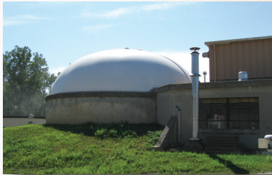
Digester Gas Holding Cover
