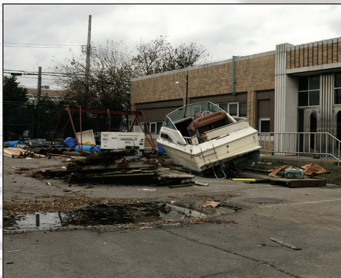
Washed up boat at the Coney Island Wastewater Treatment Plant
