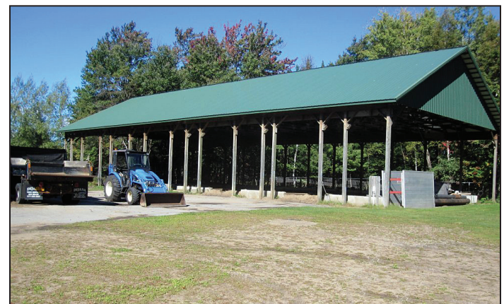
The pole barn has porous pavement drying beds and one storage bay with nonporous pavement for biosolids handling. Since 1994, the WWTP has been permitted to land apply its treated solids in May, July and September.
