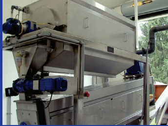
Groton NY WWTP Model 3012 DSP Screw Press
