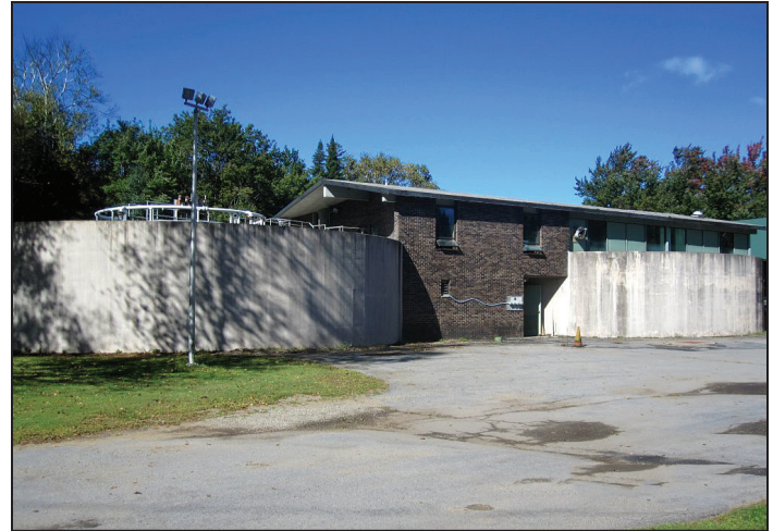
Village of Speculator WWTP's renovated Administration and Laboratory Building (left). The treatment operations facility (right) has new panels and glass enclosure for the enclosed unit as well as new coating on the outside of the circular aeration tanks.
