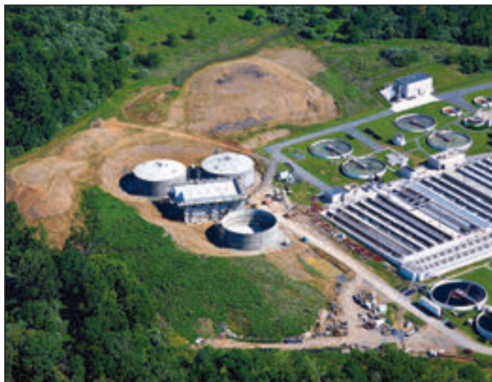
An aerial view of the construction of the FWSA Green Energy Facility, where the primary digesters are at rear of the control building and the secondary digester is in foreground.
