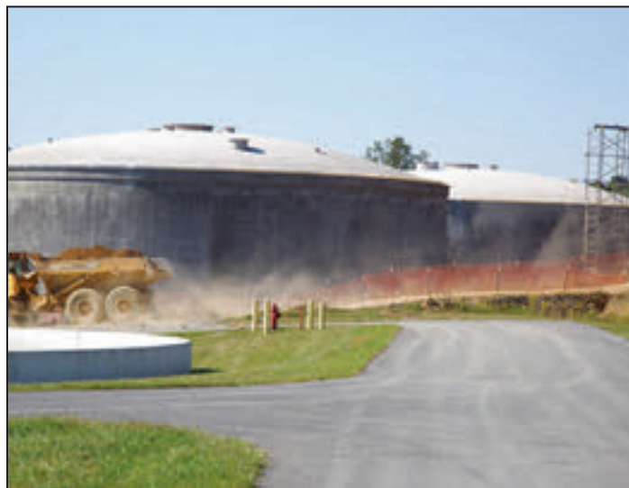
Seen here are the two 1.25 million gallon primary digesters of the new Green Energy Facility.
