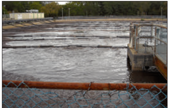
The new DO system controls the air supply in the Erie County Big Sister Creek aeration basins.
