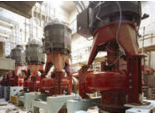
Vertical Pedestal Mounted (VPM) Dry Pit Configuration (YCC)
