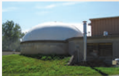
Digester Gas Holding Cover
