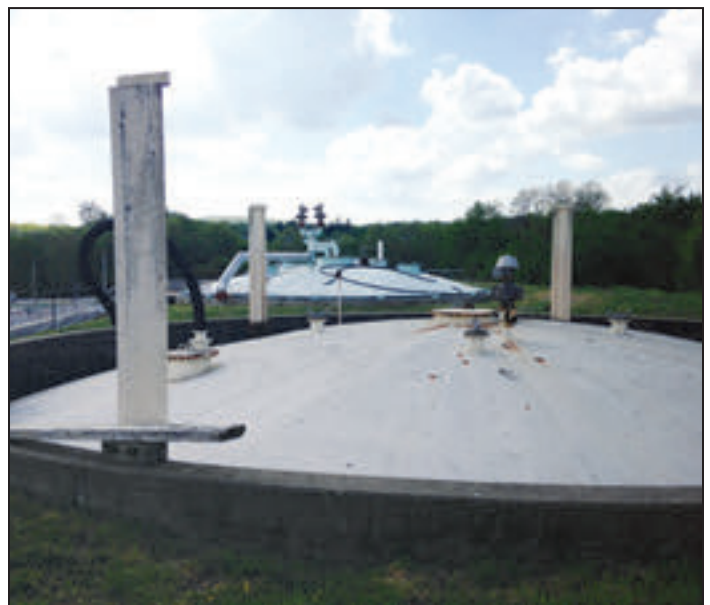
These are the existing covers of the anaerobic digesters.
