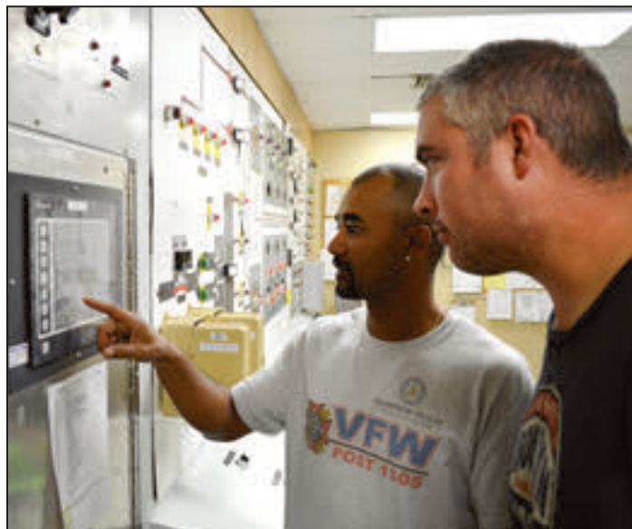
Vash Egelson (left) shows Eric Bertrand how to operate the PLC, aka SCADA system, to include clearing alarms and viewing incoming data.
