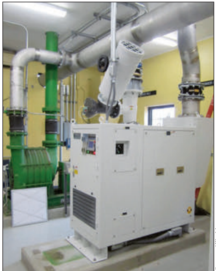
New 50 HP turbo blowers coupled with new automated DO control system will modulate blower output based on actual process demands.
