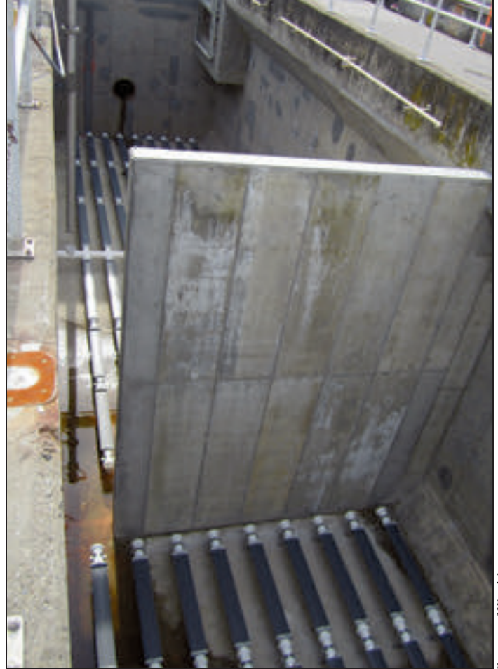
New ultra-fine bubble diffusers with an oxygen transfer efficiency of 36 percent. Also shown, new baffle wall to encourage mixing in different modes of operation (conventional, step-feed, and contact-stabilization).
