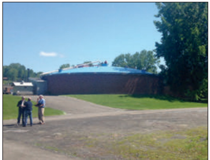
This is the proposed location of the new 1.5 million gallon primary digester, which will increase the Rome facility's organic waste receiving capabilities.
