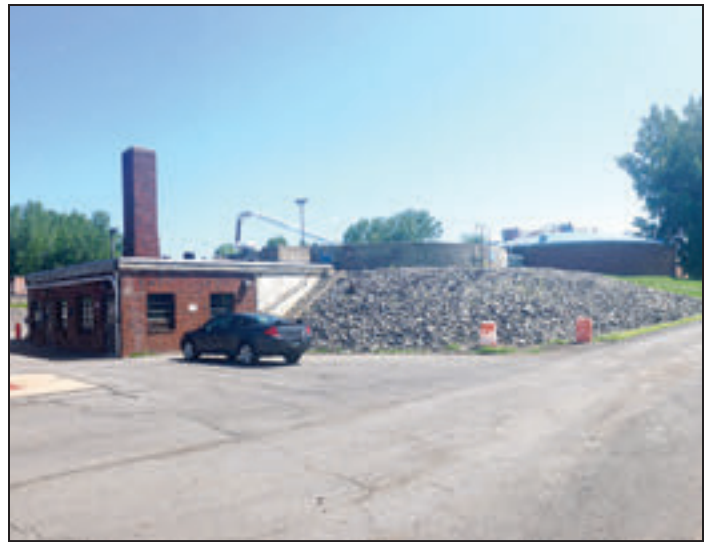
Rome's existing anaerobic digester complex is seen here, which was constructed in the 1980s.
